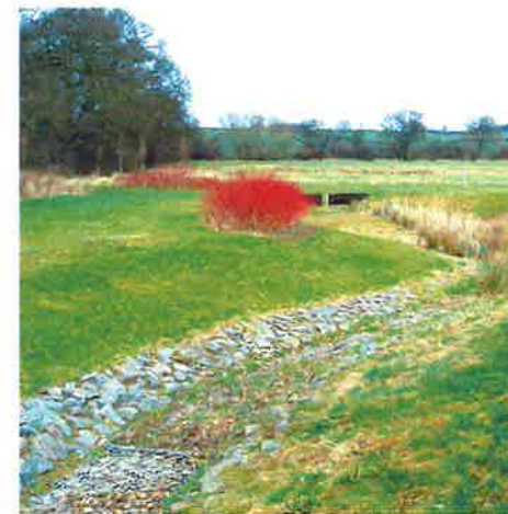
Sustainable Drainage Systems (SuDS) manage drainage as part of the landscape- providing habitats
