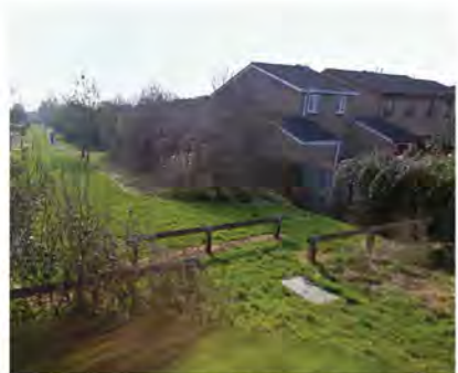
3. Greenline to Dryden Ave
