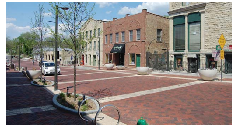
Road bands breaking-up the road culminating into geometrically planted trees aided by a raised kerb
