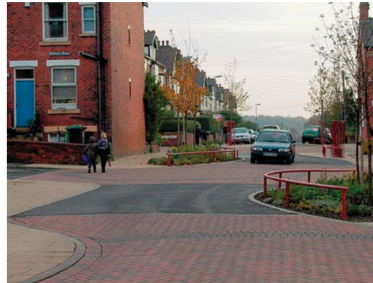
Junction raised - Distinguished by pavement
