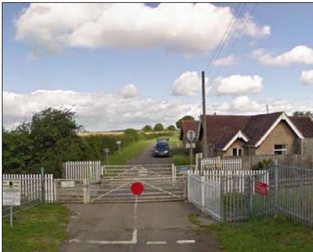
Figure 6: The Existing Mill Lane Crossing
