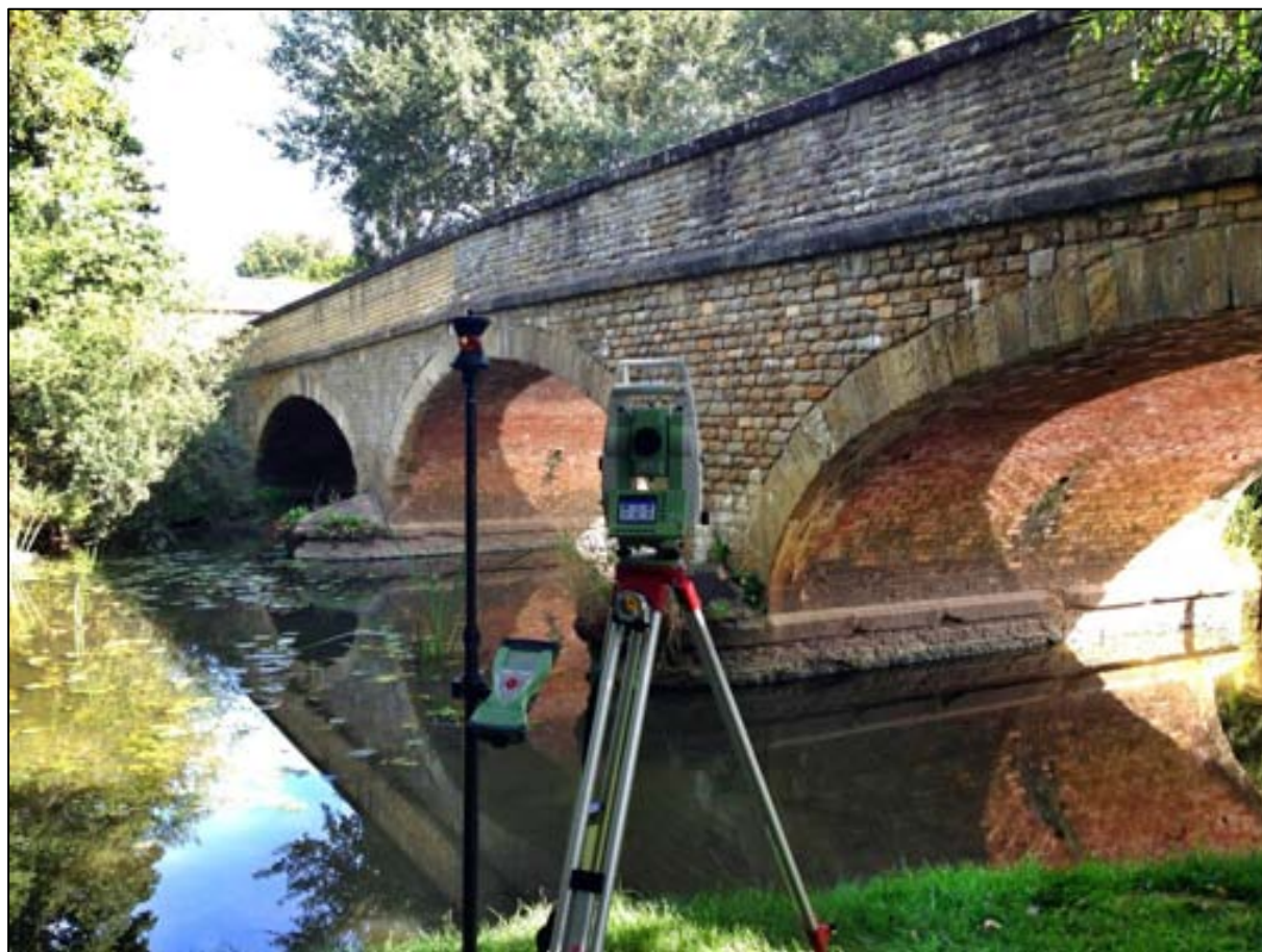
Figure 7 – B 4027 Road Bridge (Arch Bridge)
