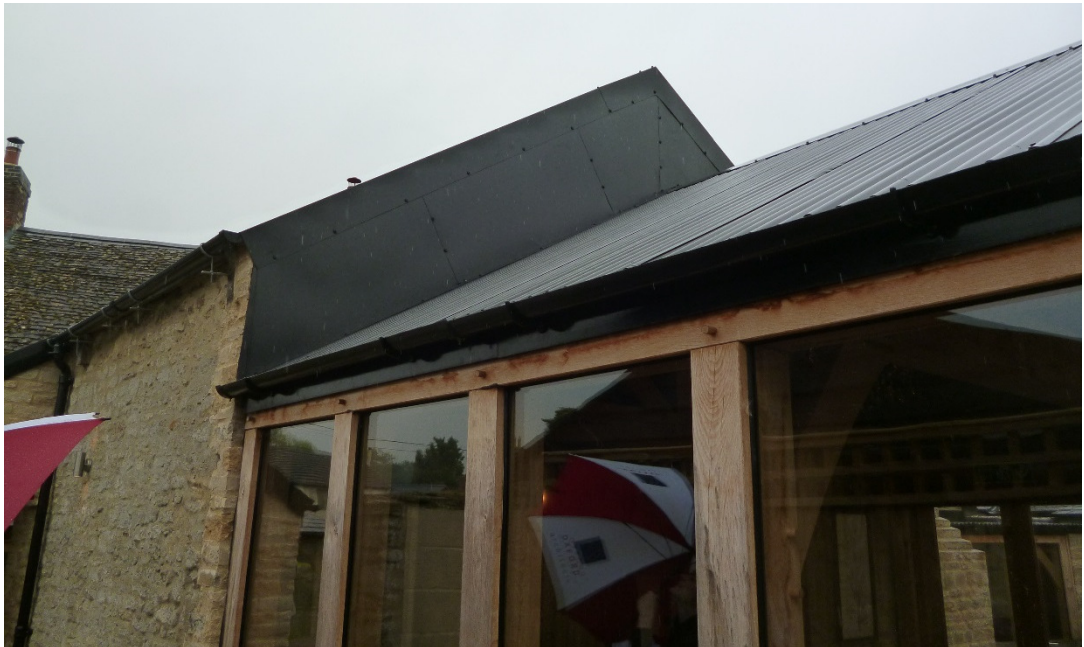
Photo 5: External view of stepped roof.
