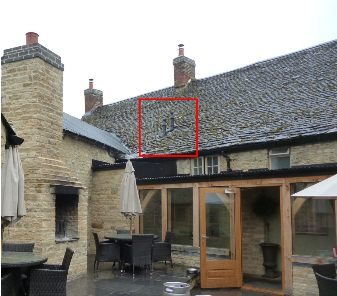
Photo 10: Relocated Flues
