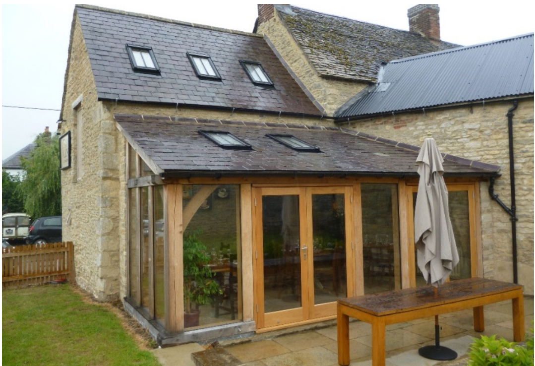
Photo 8: The roof as constructed
