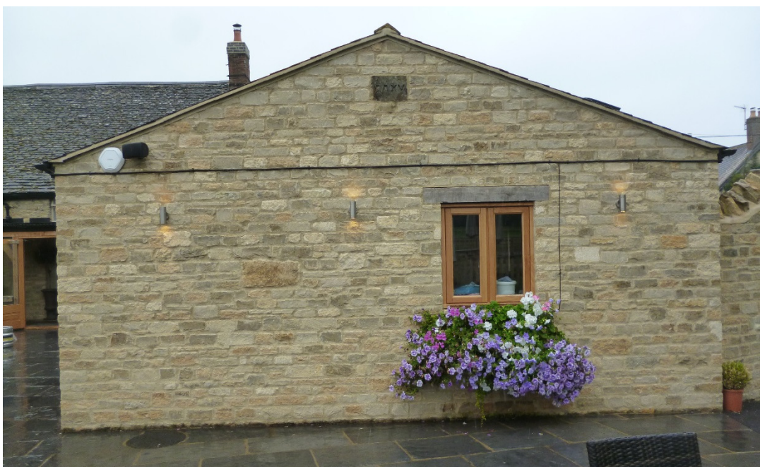
Photo 9: View of eastern gable of kitchen extension
