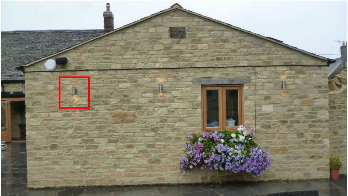
Photo 15: External lights on kitchen gable
