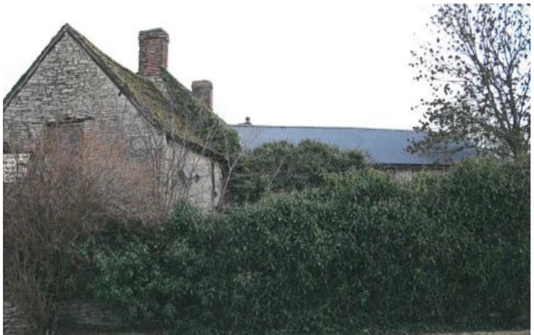
Photo 2: View of Southern Gable
