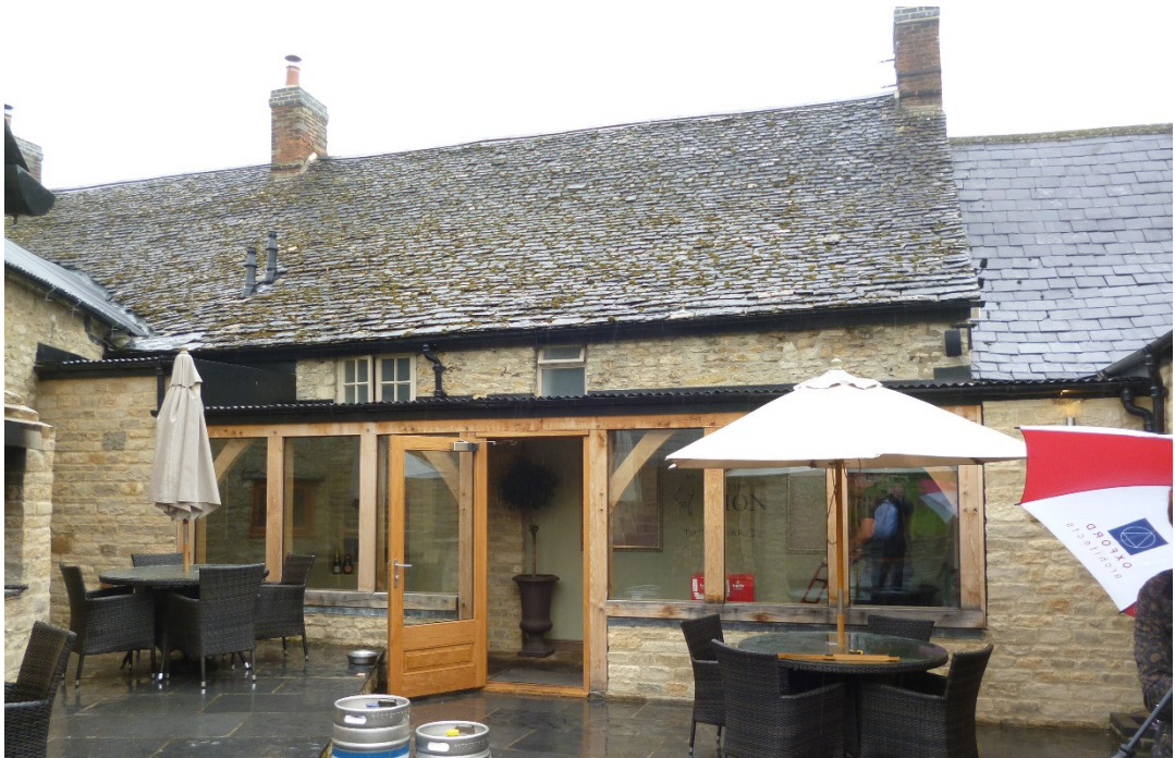
Photo 7: Photograph of new corridor link
