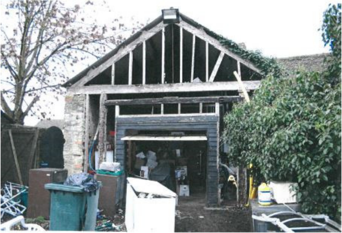
Photo 3: Gable end of barn with corrugated roof
