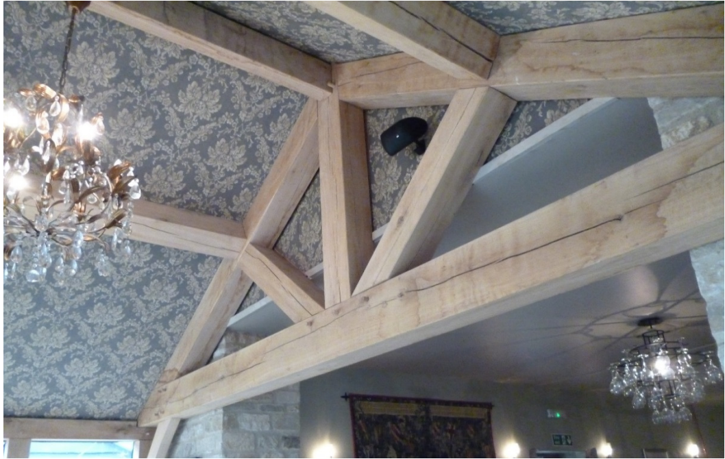
Photo 6: Internal view of stepped roof
