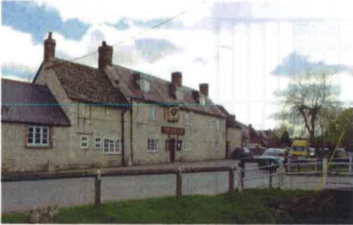
Frontage of Pub – Including bridge and Wendlebury Brook opposite
