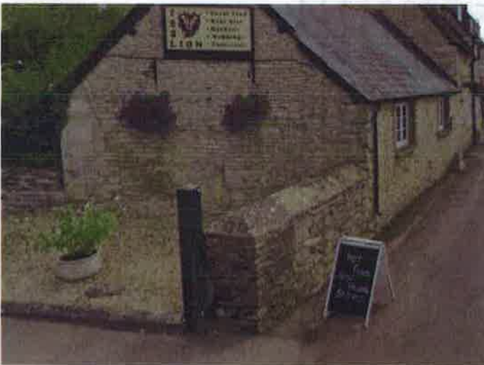
Rain Water Down Pipe discharging to road
