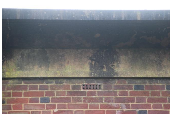
16. Concrete eaves and smaller air brick type
