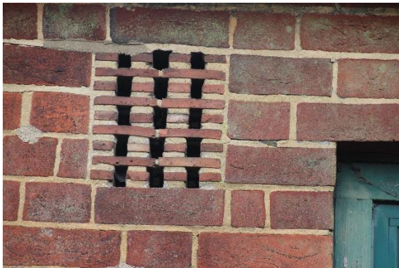
15. Close-up of large air brick type
