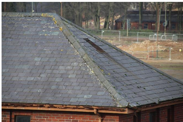
4. Air Vent on Building 485
