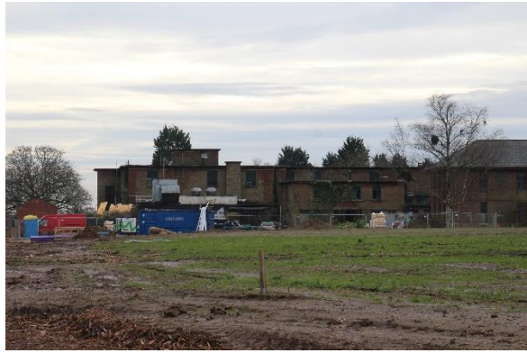
10. Building 488 from the north
