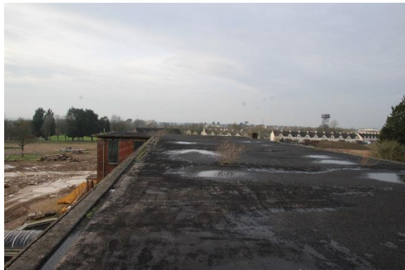
12. Felt flat roof looking east
