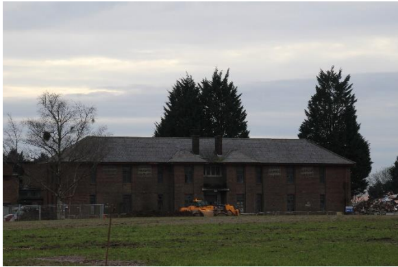
1. Building 485 from the north
