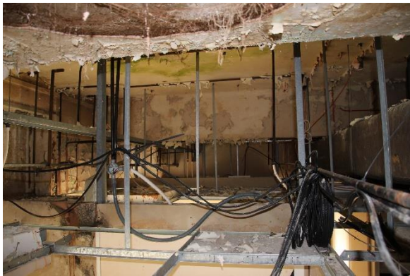
13. Space above false ceiling in two storey section
