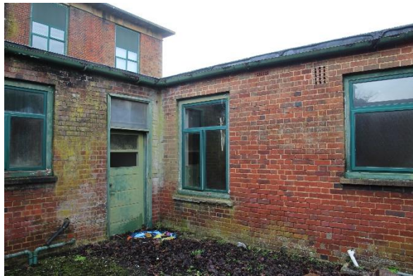
14. Two types of air brick in courtyard of 488
