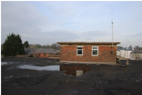
11. Felt flat roof on Building 488
