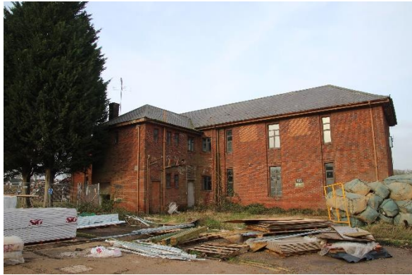
2. Building 485 from south-east
