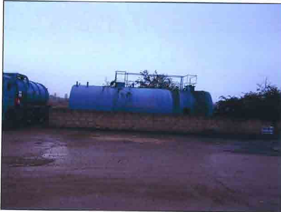
Plate 5: Oil storage in Grundon compound.
