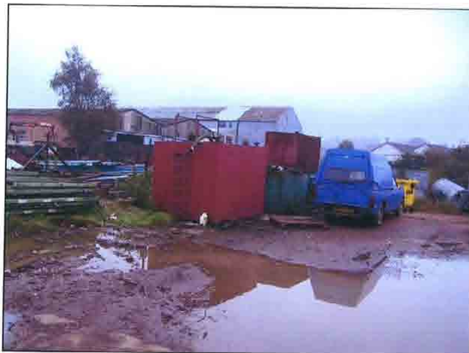
Plate 6: Redundant oil tank storage.
