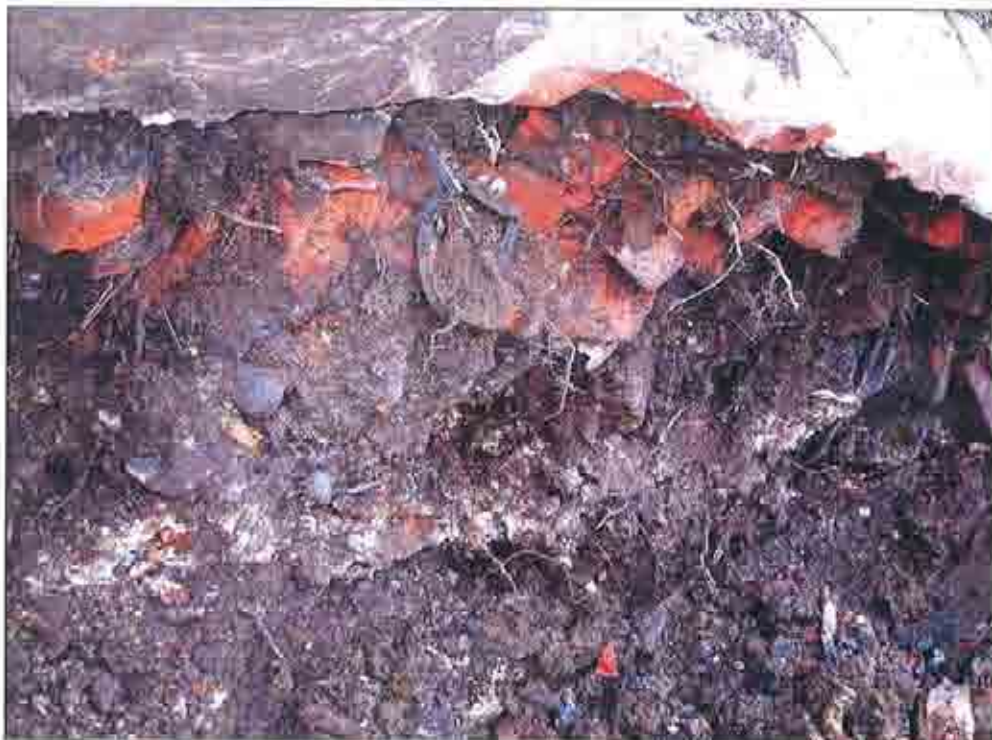
Plate 28: Layer of potentially fibrous asbestos (0.3m thick x 1.8m long) encountered at 1.2m bgl
