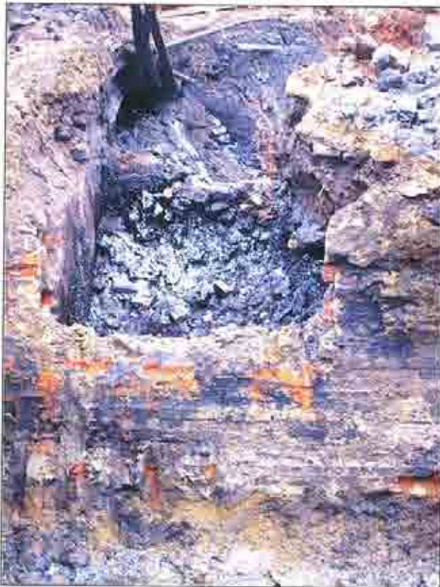
Plate 19: Western wall of Chamber 3 with significant volume of tarry residues
