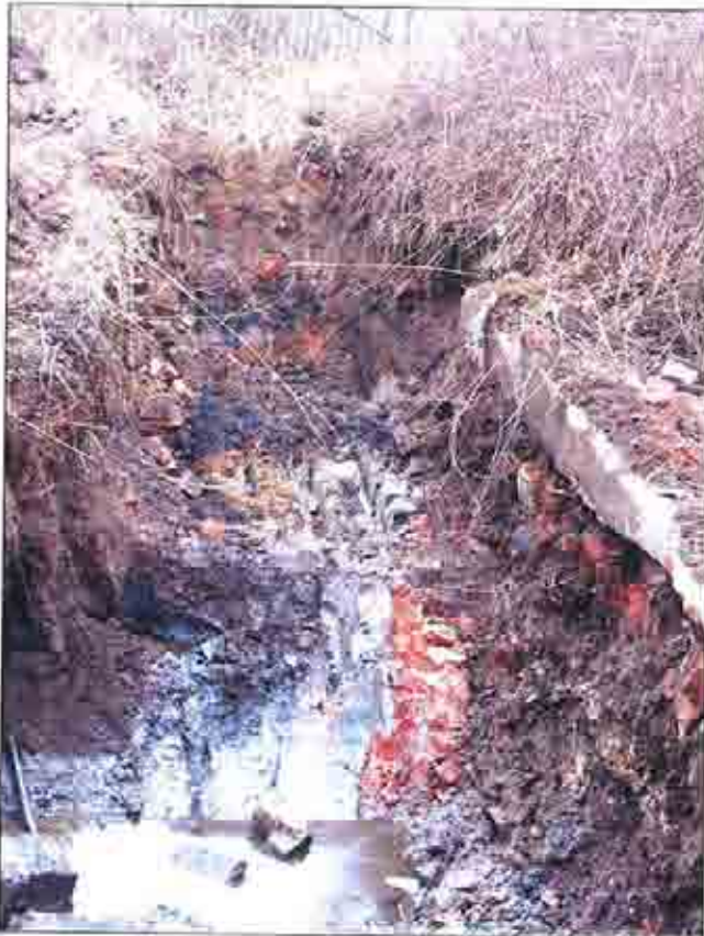
Plate 31: Contaminated water rising to surface from redundant pipework on the northeastern face of trial trench (noxious ammonia odour)
