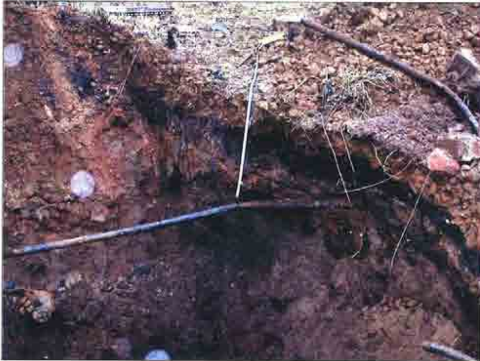
Plate 3: 25mm Ø iron pipe located in made ground, trending northwest/southeast
