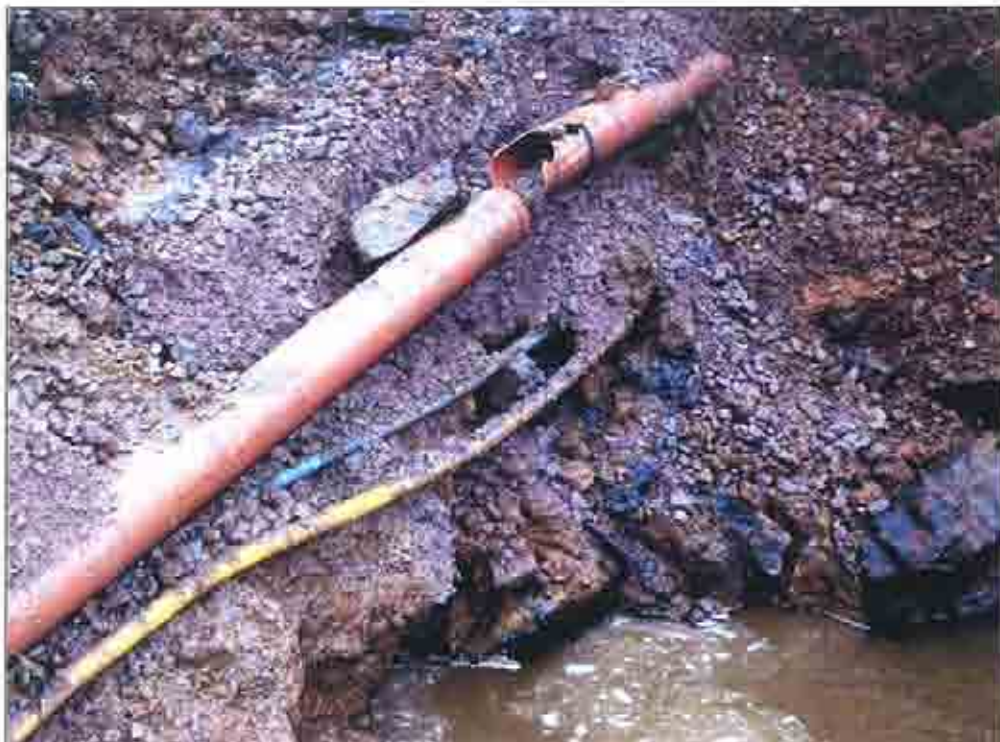
Plate6: 3No services encountered on northwestern face of trial pit
