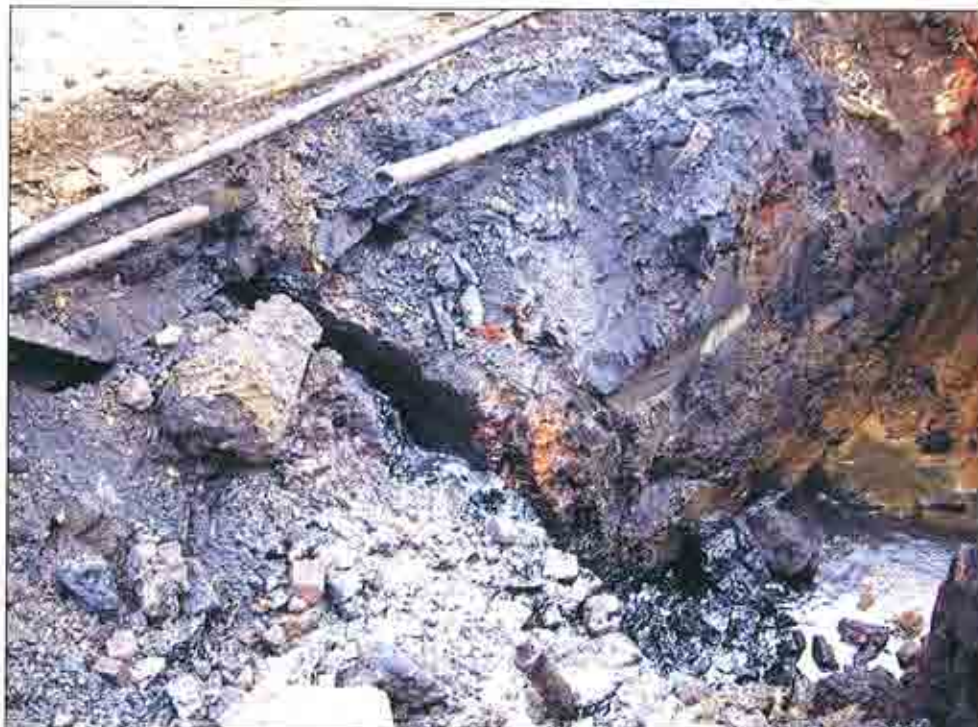
Plate 16: Southern wall of Chamber 1 with significant volume of tarry residues
