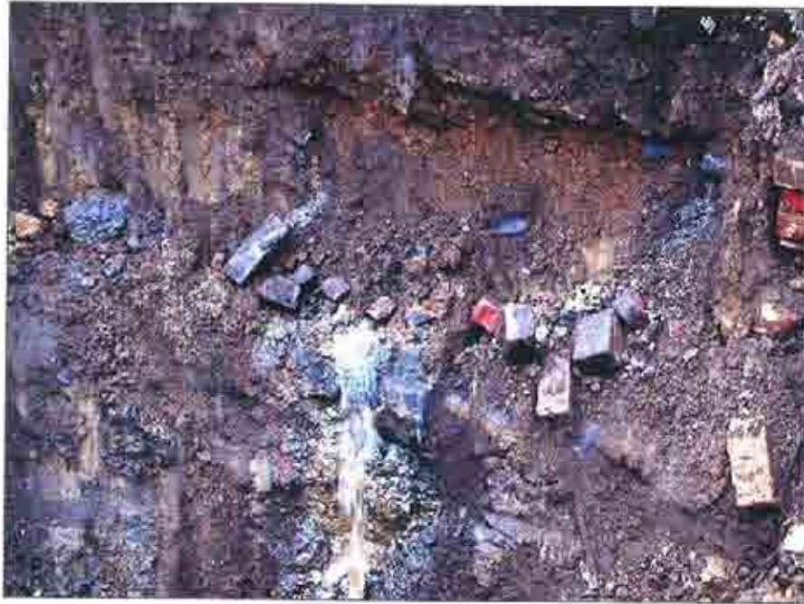
Plate 31: Contaminated water rising to surface from redundant pipework on the northeastern face of trial trench (noxious ammonia odour)
