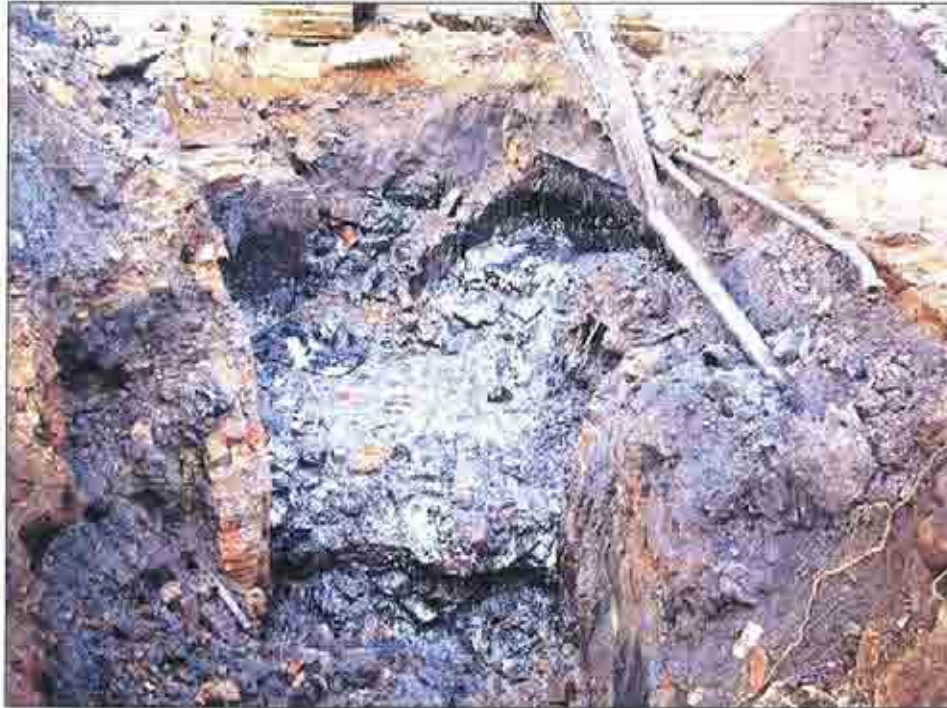
Plate 17: Western wall of Chamber 1 with significant volume of tarry residues
