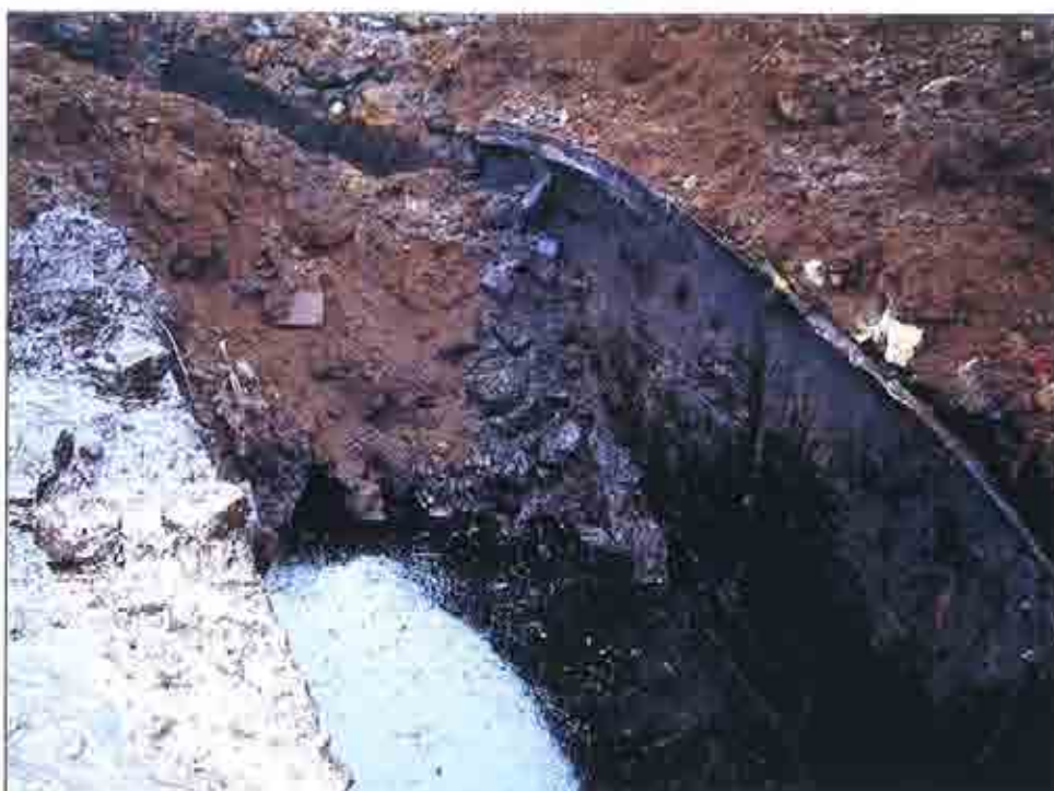
Plate 26: Contaminated residues contained in vessel with concrete pad to the north
