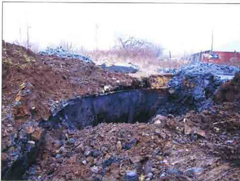
Plate 22: Riveted iron panels of underground vessel
