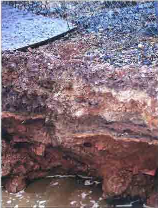
Plate 5: Rapid inflow of groundwater from Transco compound to southeast
