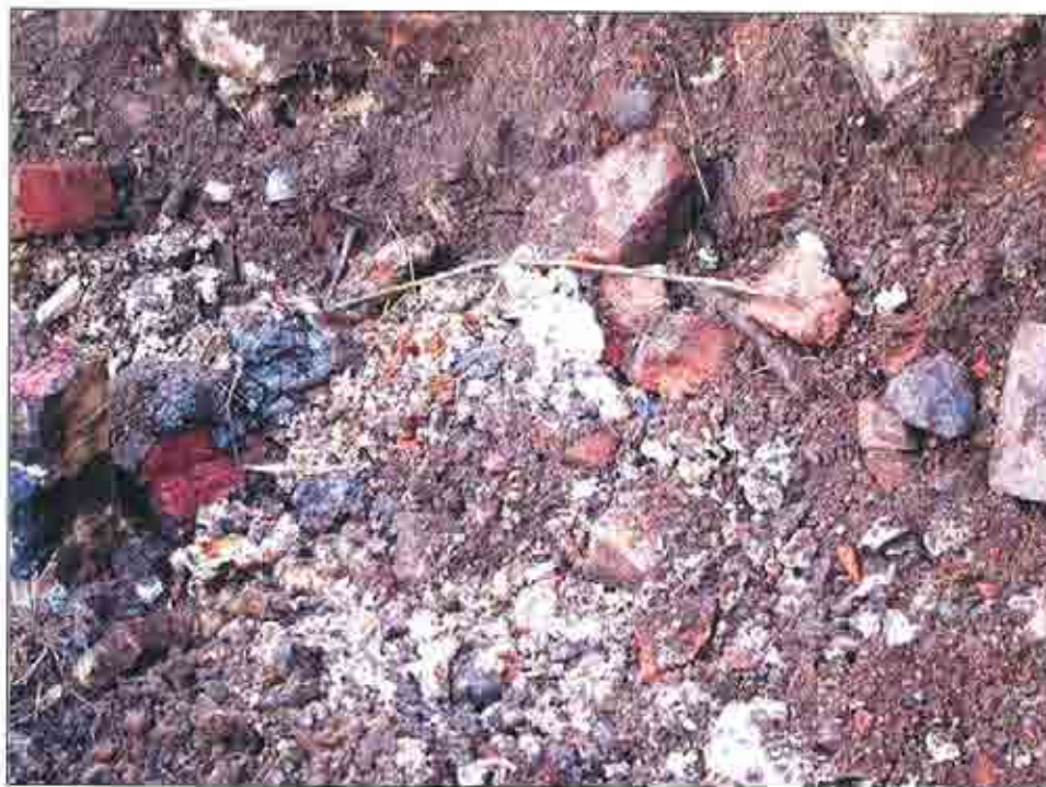
Plate 29: Close-up of potential asbestos containing material
