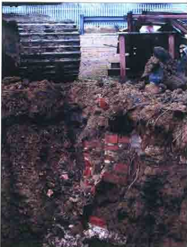
Plate 3: 25mm Ø iron pipe located in made ground, trending northwest/southeast
