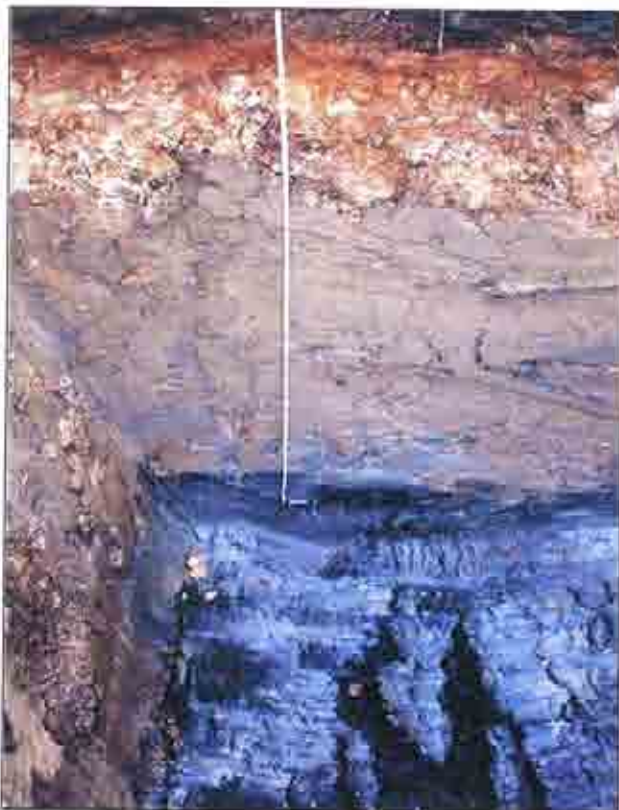
Plate 34: Significant contamination of alluvium beneath existing Grundon carpark area
