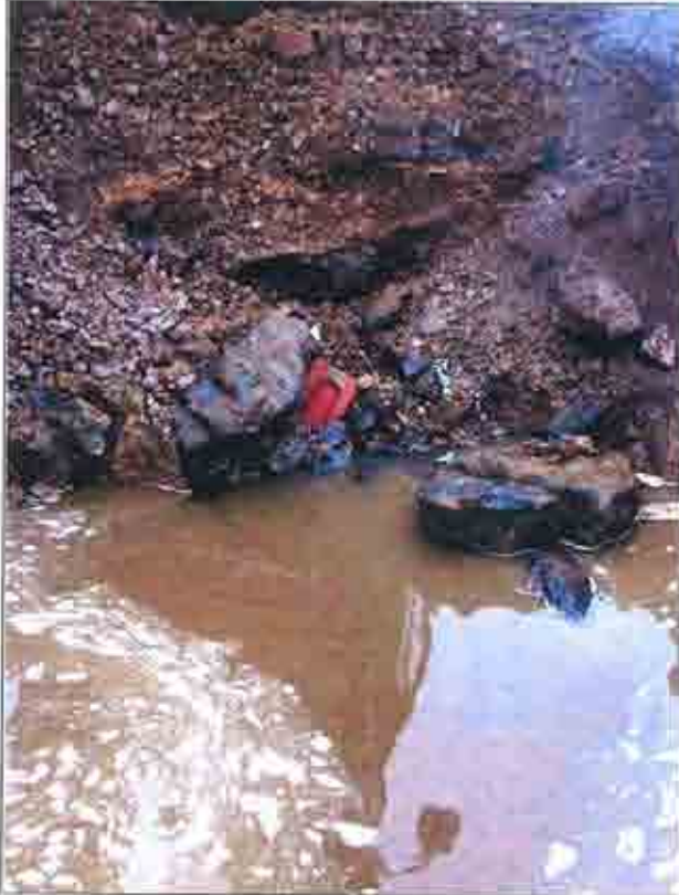
Plate 7: Rapid inflow of groundwater from Transco compound to southeast
