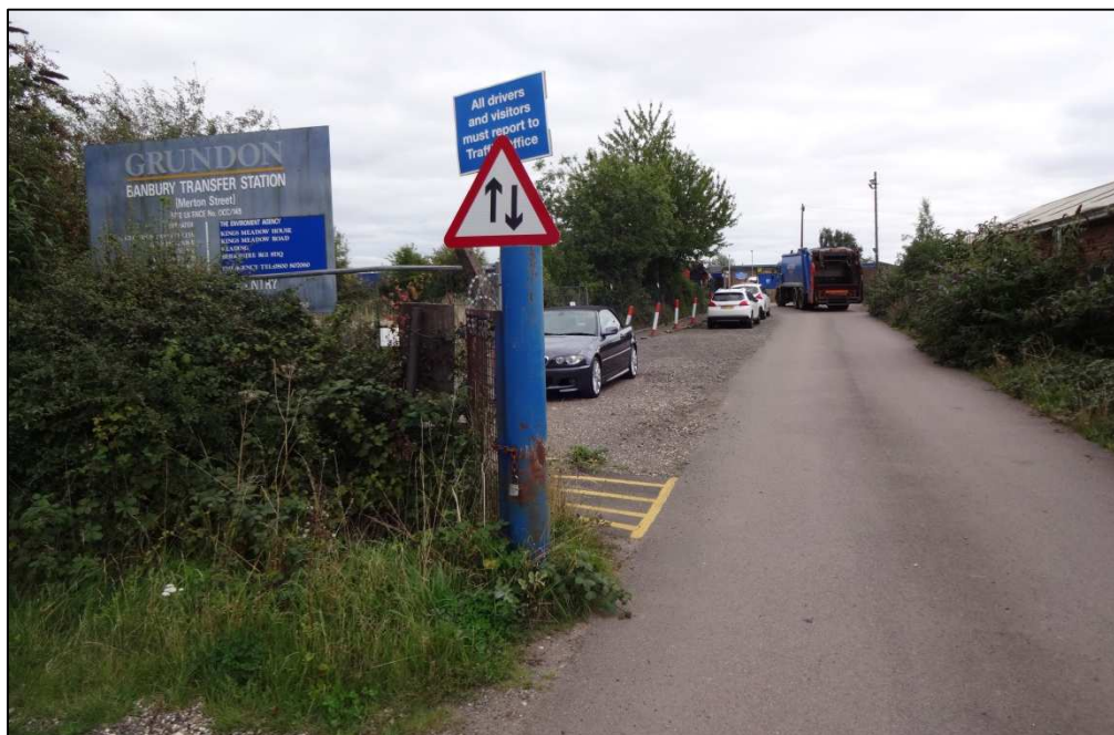
Figure 2.2: View south-east at site entrance
