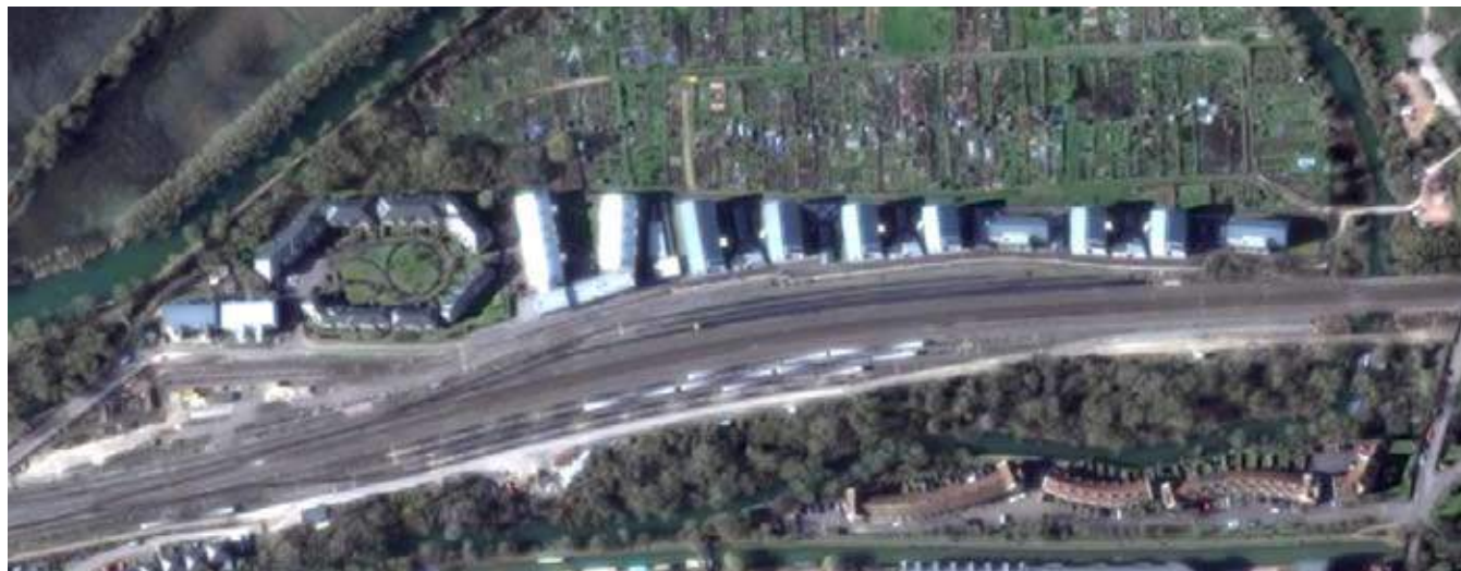
Example of flanking development onto railway - Rodger Dudman Way, Oxford
