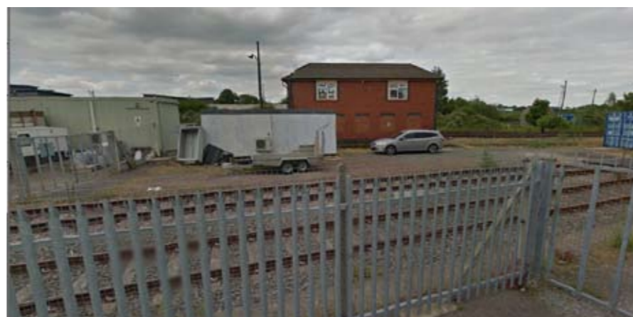
Signal box viewed from the south
