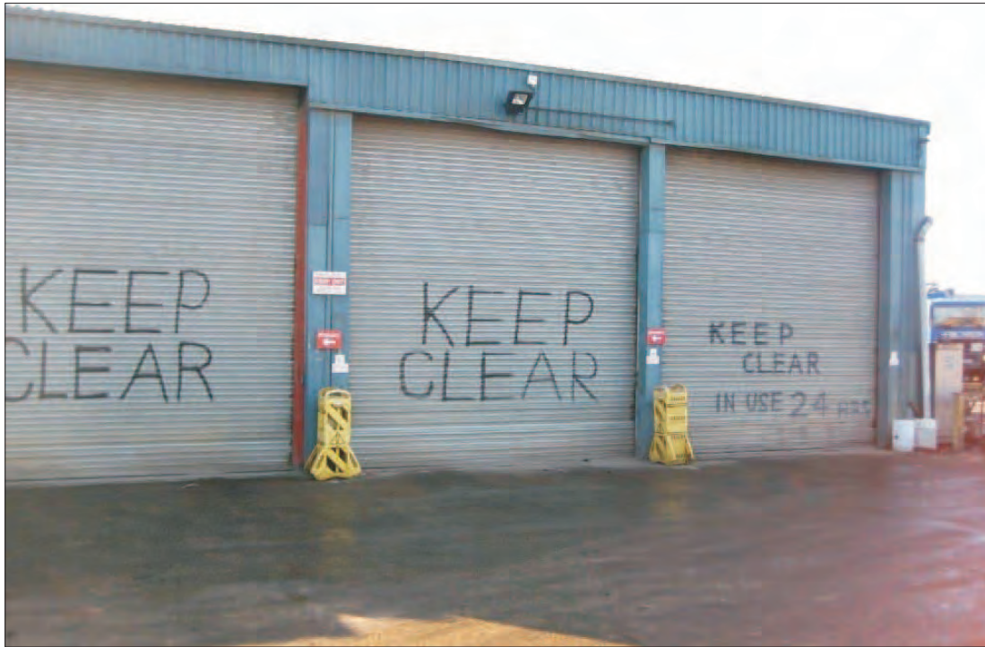
PHOTOGRAPH 7: BUILDING B3 VIEWED FROM THE NORTH
