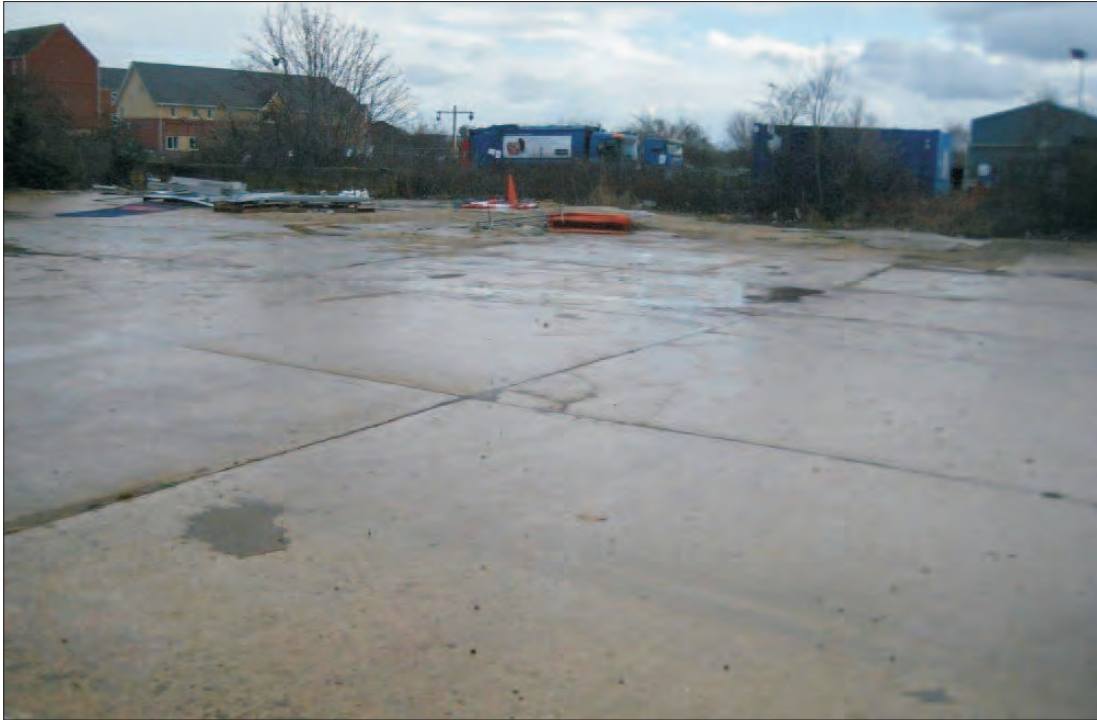
PHOTOGRAPH 1: RECOLONISING GROUND / HARDSTANDING
