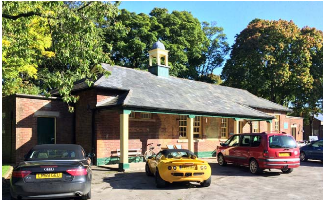
Fig 5. View of the guard house front elevation, showing the covered canopy.
