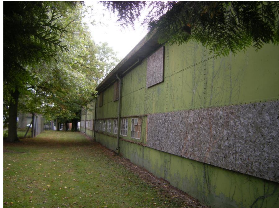
Rear elevation from south east
