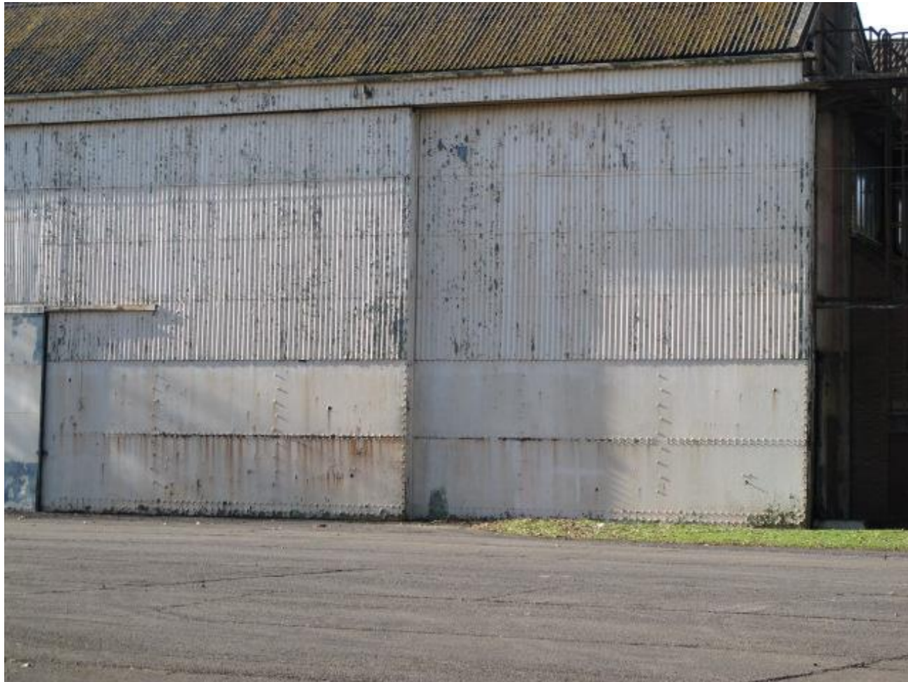
Traditional corrugated iron cladding on Building 79
