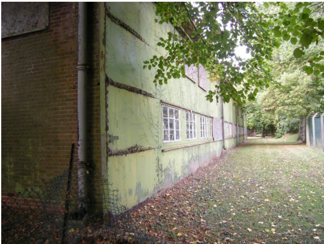
Rear elevation from north west
