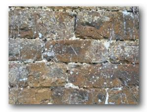
The photograph to the right is a close-up of the sample panel now constructed on site. This stone has been carefully chosen to use sizes to match existing and has been hand cut/formed to pick up the suggested tooling marks outlined by the conservation officer.
