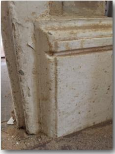
The photograph above shows the profile end of the ground floor skirting board. This is the same skirting as shown in the left-hand picture, and shows the junction detailing at a door frame location.
