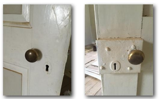
Below is an image of a new brass door lock system, if my client is not successful finding reclaimed handles to match, then a new handle set as per below is to be used for each new door opening, this is to be purchased from Broughtons of Leicester.
