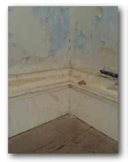
The above skirting board is used within the existing ground floor sitting room and dining room, and is noted as being approximately 8 inches high. This profile in detail is to be used for any replacement/ repair skirting board or new skirting boards throughout the ground floor.
