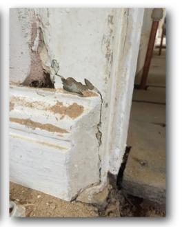
The photograph above shows the skirting board at first-floor level, and this is the same profile as the ground floor, but with a shallower overall depth. This profile in detail is to be used for any replacement/repair of skirting board or new skirting boards throughout the first floor.
