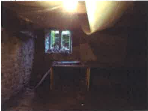
Plate 7: Cellar beneath house
