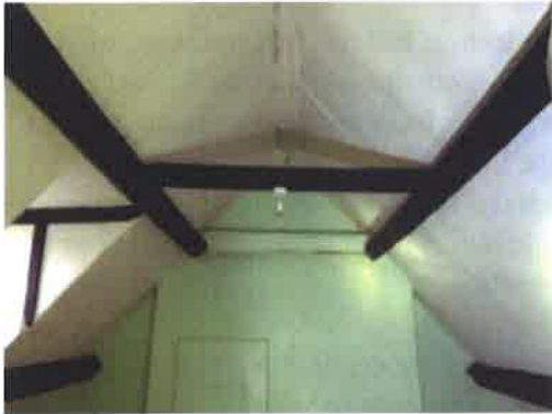
Plates 5 and 6. Third storey interior within the main house; showing the west room (left) and east room (right); the east room has a false ceiling, installed at the level of the purlins, with a small void above understood to contain thick insulation material.
