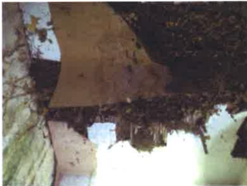
Plates 9 and 10: Interior areas of outbuilding; showing extensive ivy ingress into the south (left) and north (right) roof spaces.
