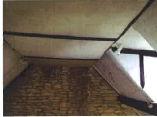
Plates 5 and 6. Third storey interior within the main house; showing the west room (left) and east room (right); the east room has a false ceiling, installed at the level of the purlins, with a small void above understood to contain thick insulation material.
