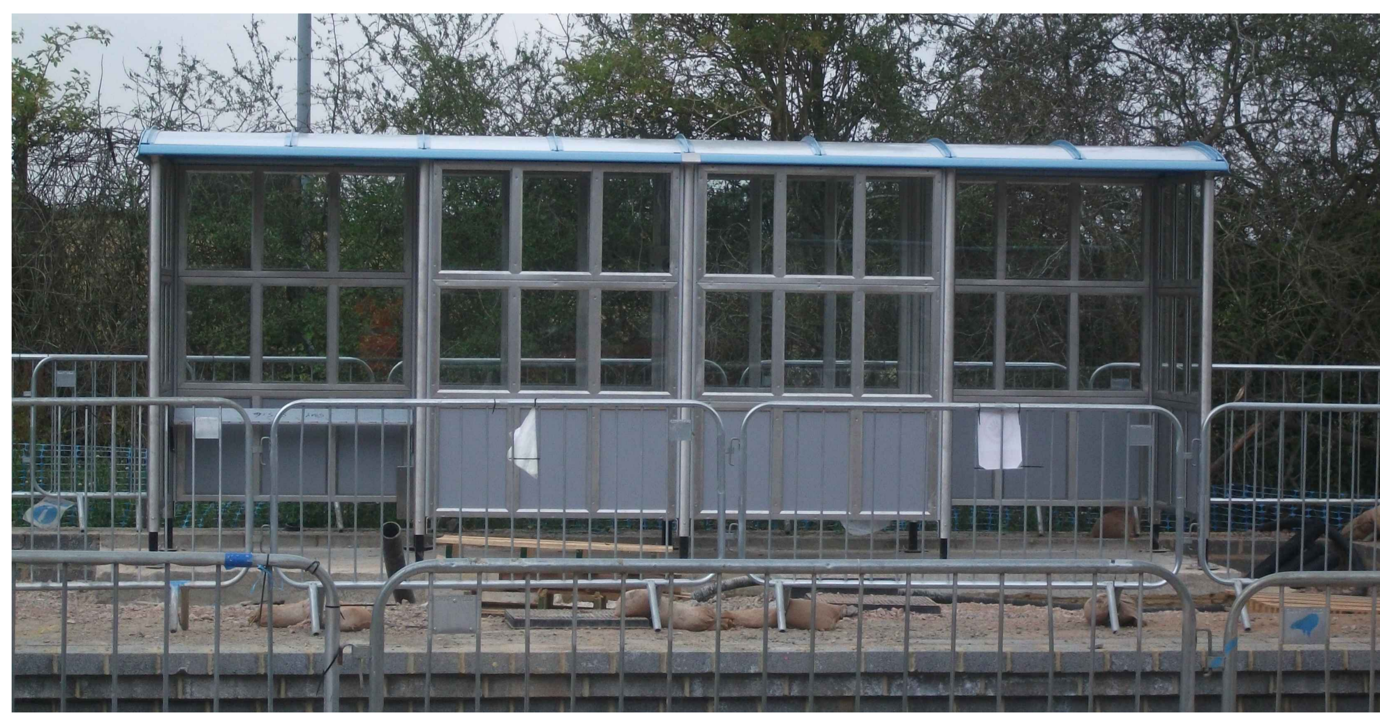
PHOTO OF PLATFORM SHELTER
