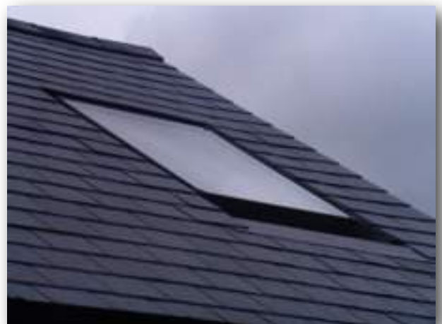
The above photograph shows a recently installed “Neo” rooflight flush fitting within a slate roof and clearly shows how simple the glass panel looks
