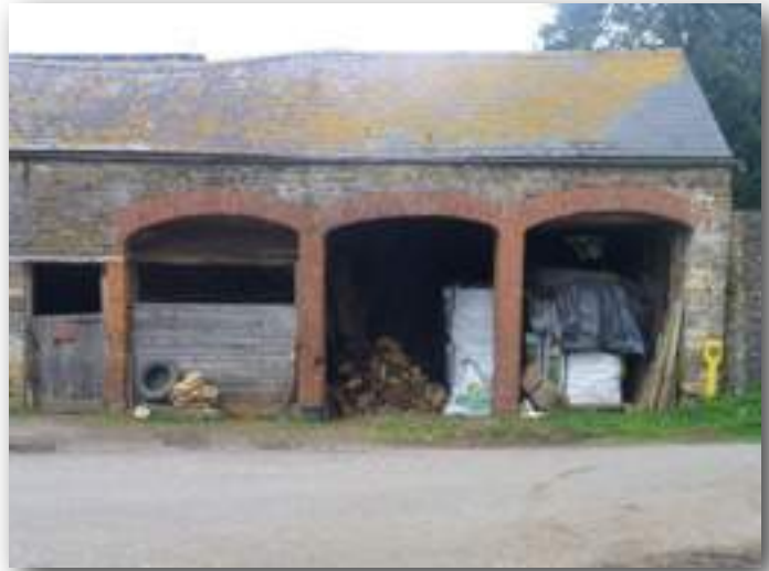
This is a photograph showing the brick arches clearly visible from the road frontage in one of the barns at Temple Mill.
