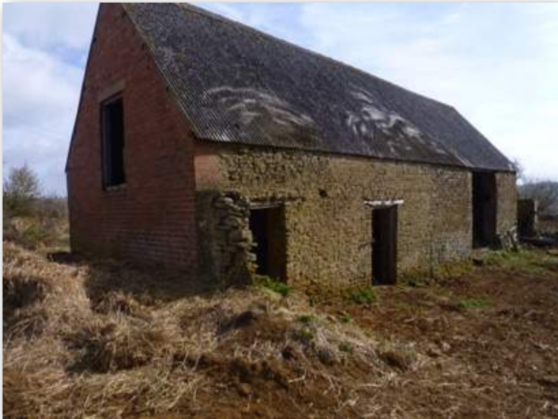
Photograph of the south elevation showing the remaining element of part of the courtyard wall and the brickwork west end gable
