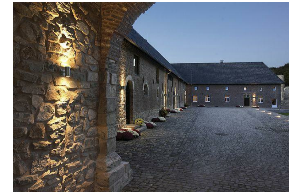
The photograph above shows a typical example of the wall mounted up and down lighting that we propose to fix to the barn conversion in the approximate locations as shown
