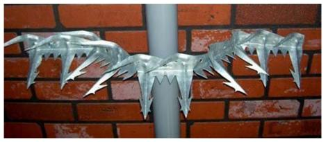
Secured to drainpipes and telegraph poles these anti-climb razor spike collars are intended to prevent people from climbing but would also prevent cats from climbing the buildings and gaining access across the fence line.
