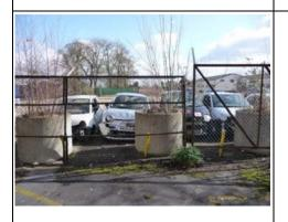
Chain link fence with concrete supports approx. 1.8m high with 45° overhang of either barbed wire strips or razor wire strips.
