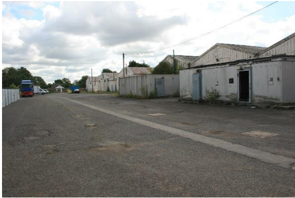
1. Northern end of site and buildings
