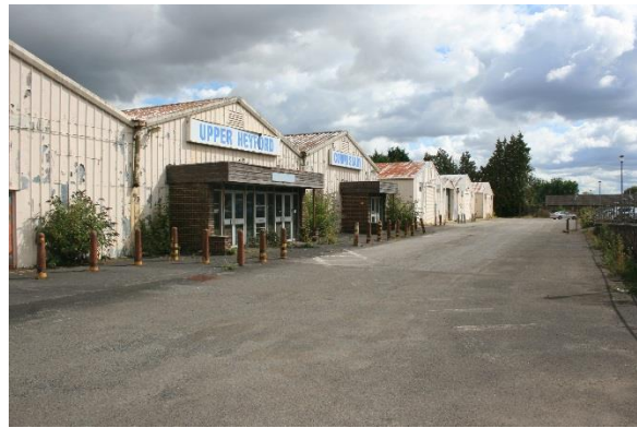
2. Southern end of buildings
