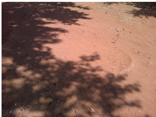
Photograph 3: Exposed and damaged roots
