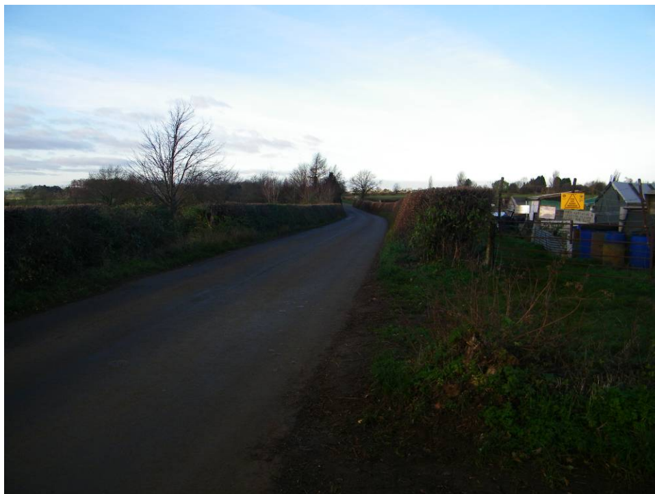
FIGURE 9: WYKHAM LANE (FORMER ROMAN ROAD), FROM THE EAST
