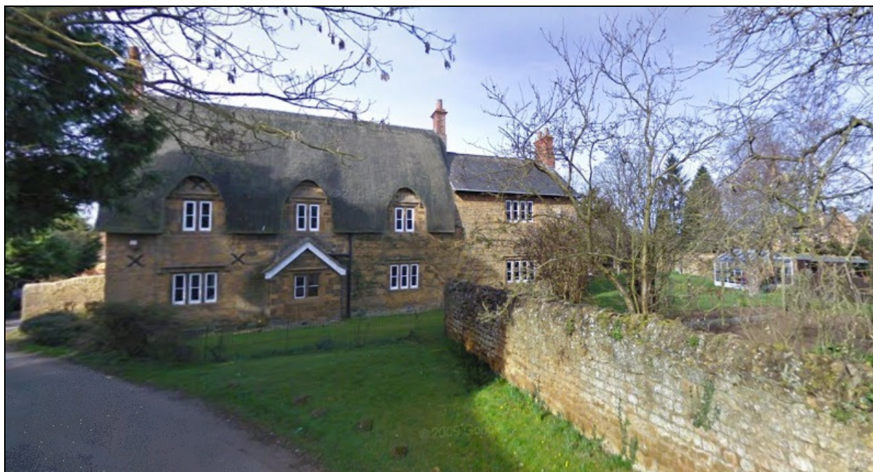
Figure 11: Grade II Listed Old Barn House, looking north-west
