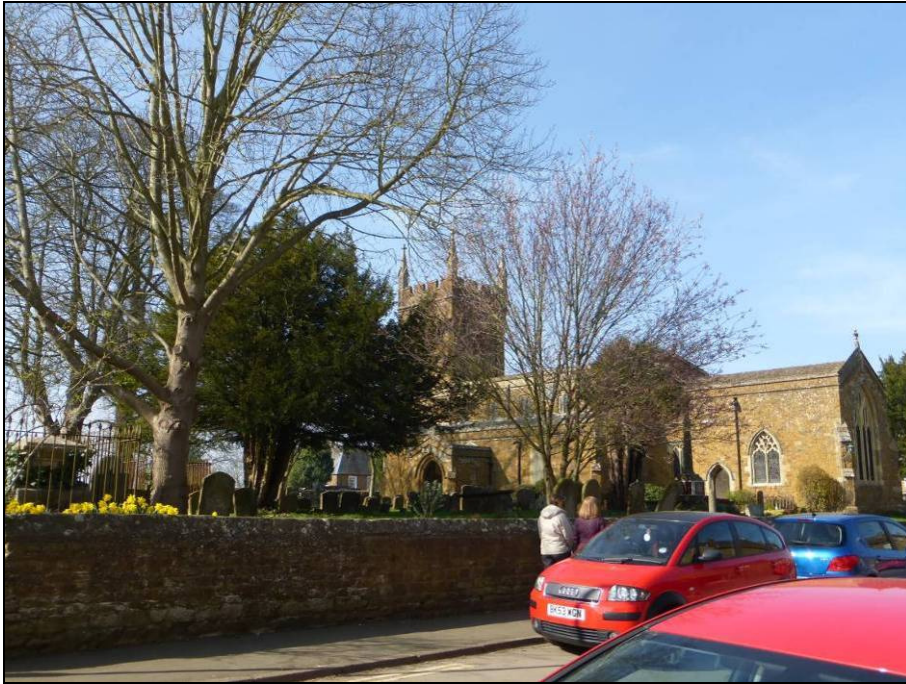
Figure 8: Grade II* Church of St John the Baptist, Bodicote, looking north-west
