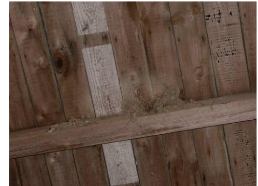
Figs. 18 & 19 Timber sarking lined roof of stable block
