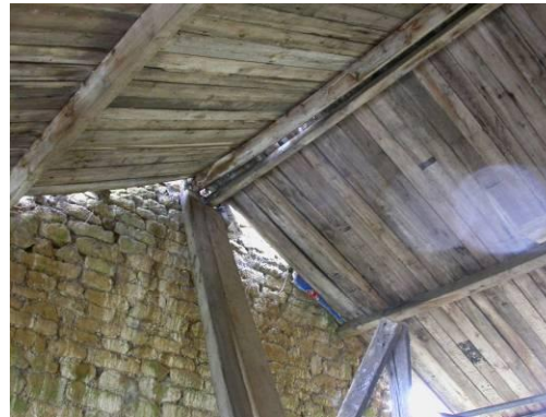
Figs. 18 & 19 Timber sarking lined roof of stable block
