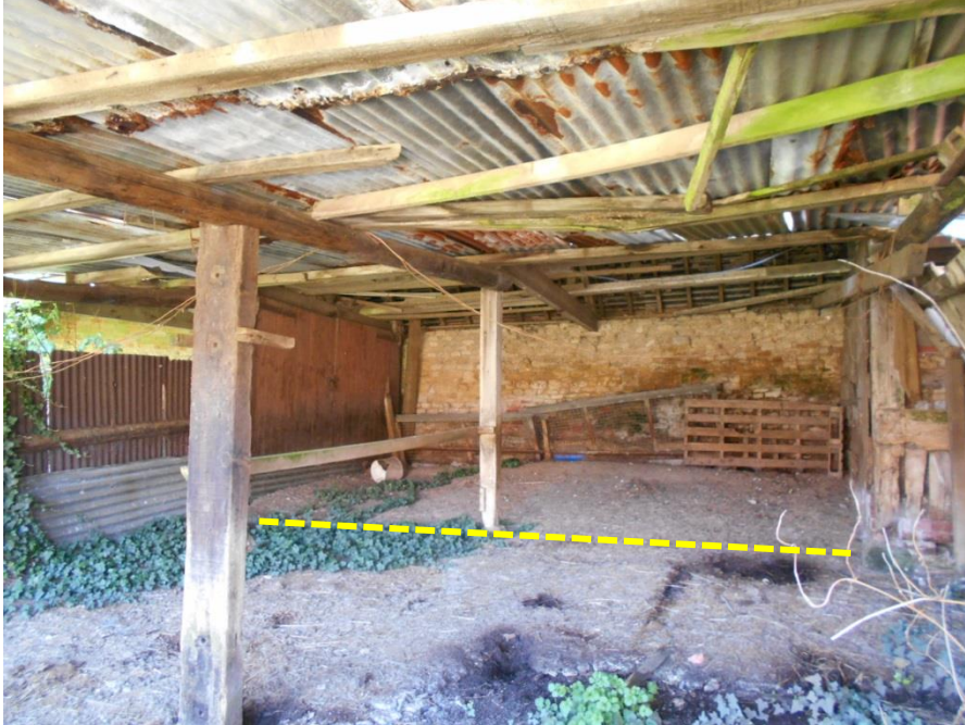
Fig 7: Building 3 interior, looking south into Building 2 (old open front is dashed)
