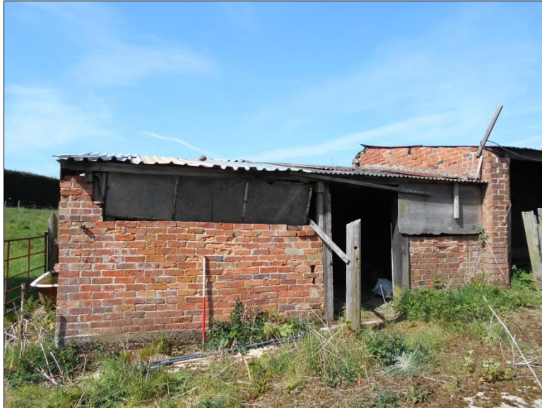
Fig 10: The southern half of Building 5, looking west; scale 1m; the footpath can be seen on top of the rise at far left
