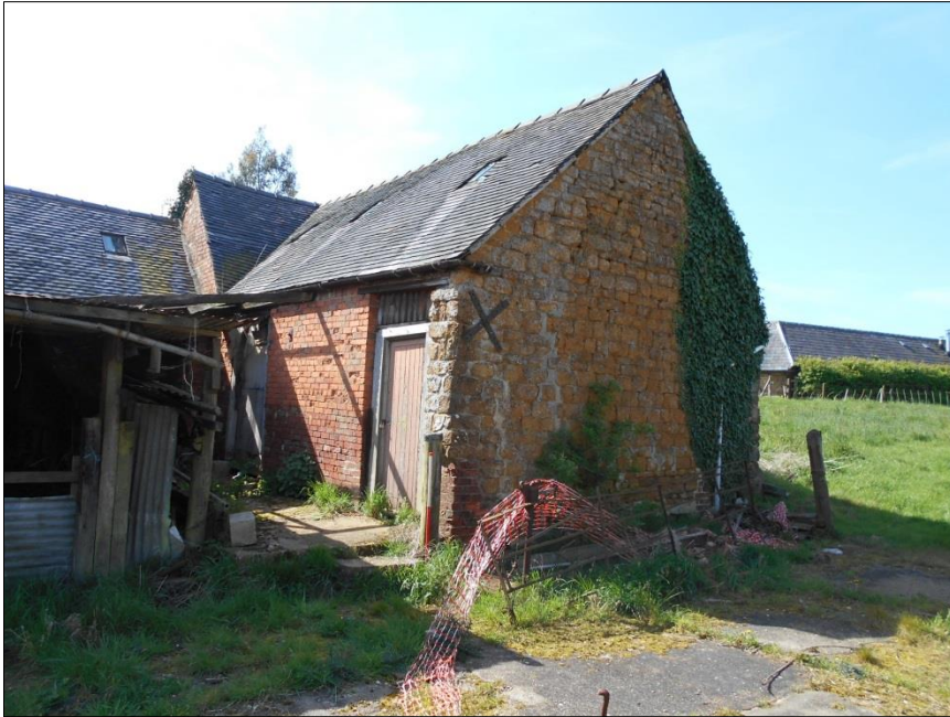
Fig 8: Building 4, looking south-west; scale 1m
