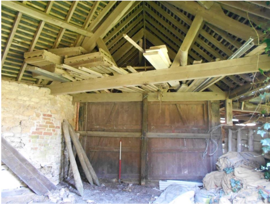
Fig 5: Building 2 interior, looking west at the roof angle; scale 1m
