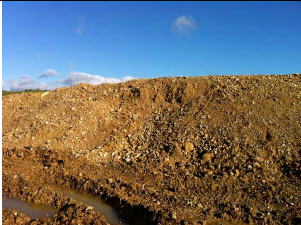
41. 07/02/14 – B581- Site generated recycled aggregate
