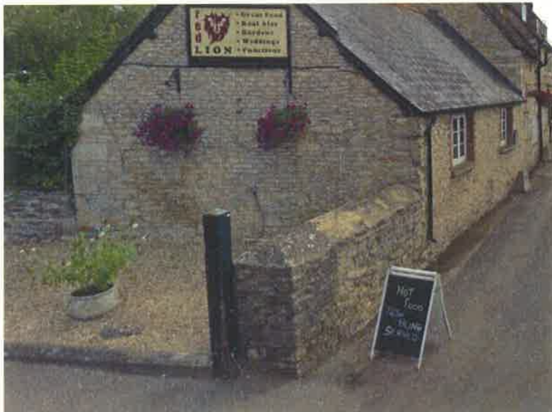
Rain Water Down Pipe discharging to road
