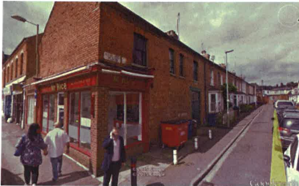
Figure 4 : Corner view of Mr. Rice and Newline Place
