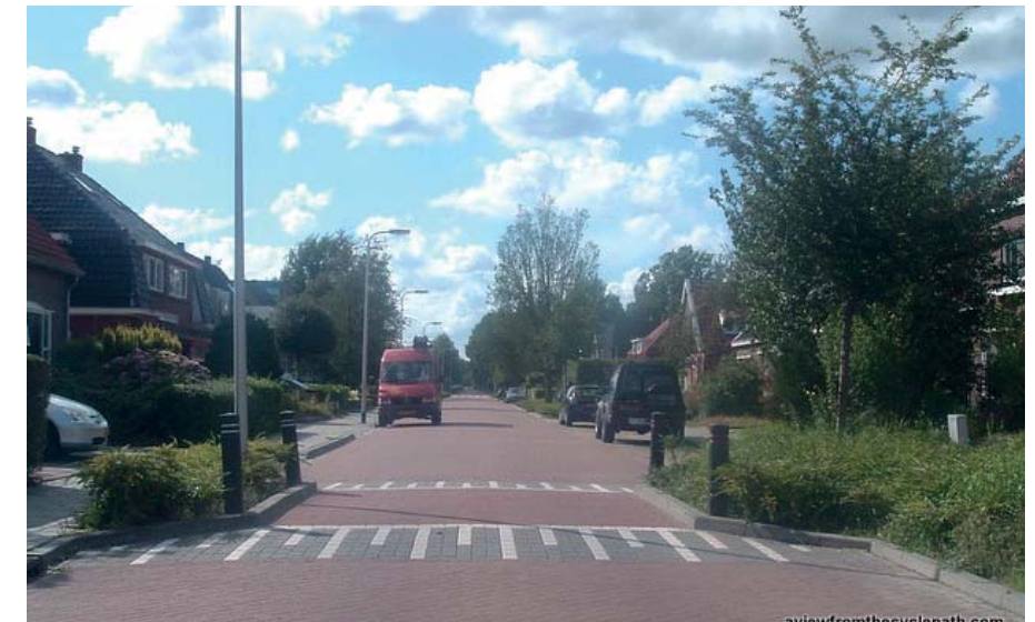
Traffic calming surfaces combined with on-street parking
