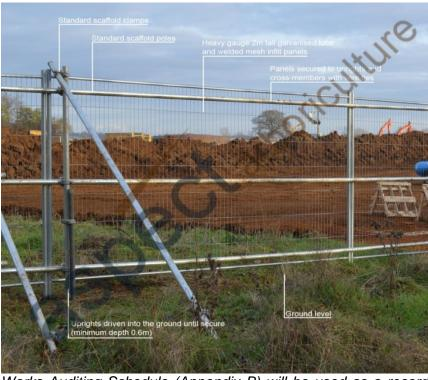
Plate.1 Default Protective Barrier Specification
