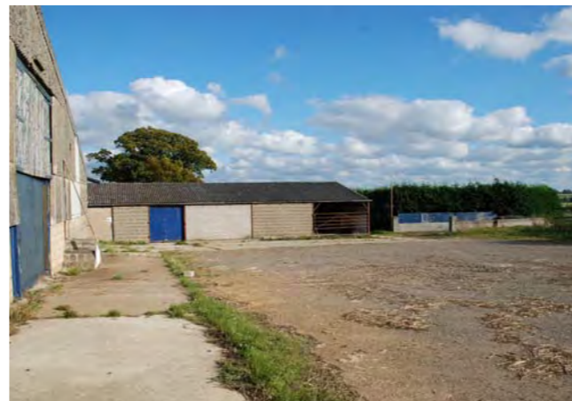
7. Existing yard looking east
