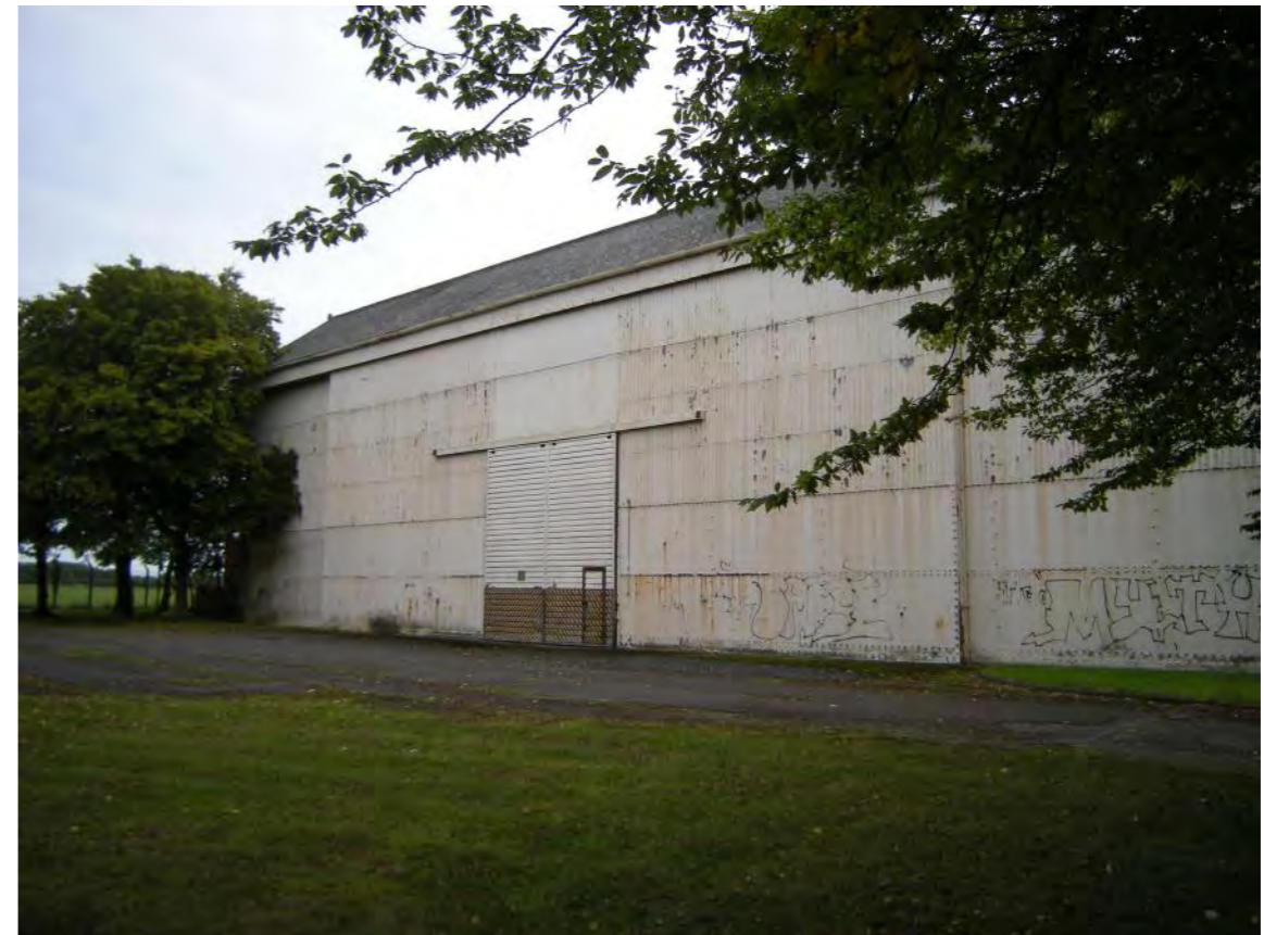
Fig 21: the sliding end doors of Building 79
