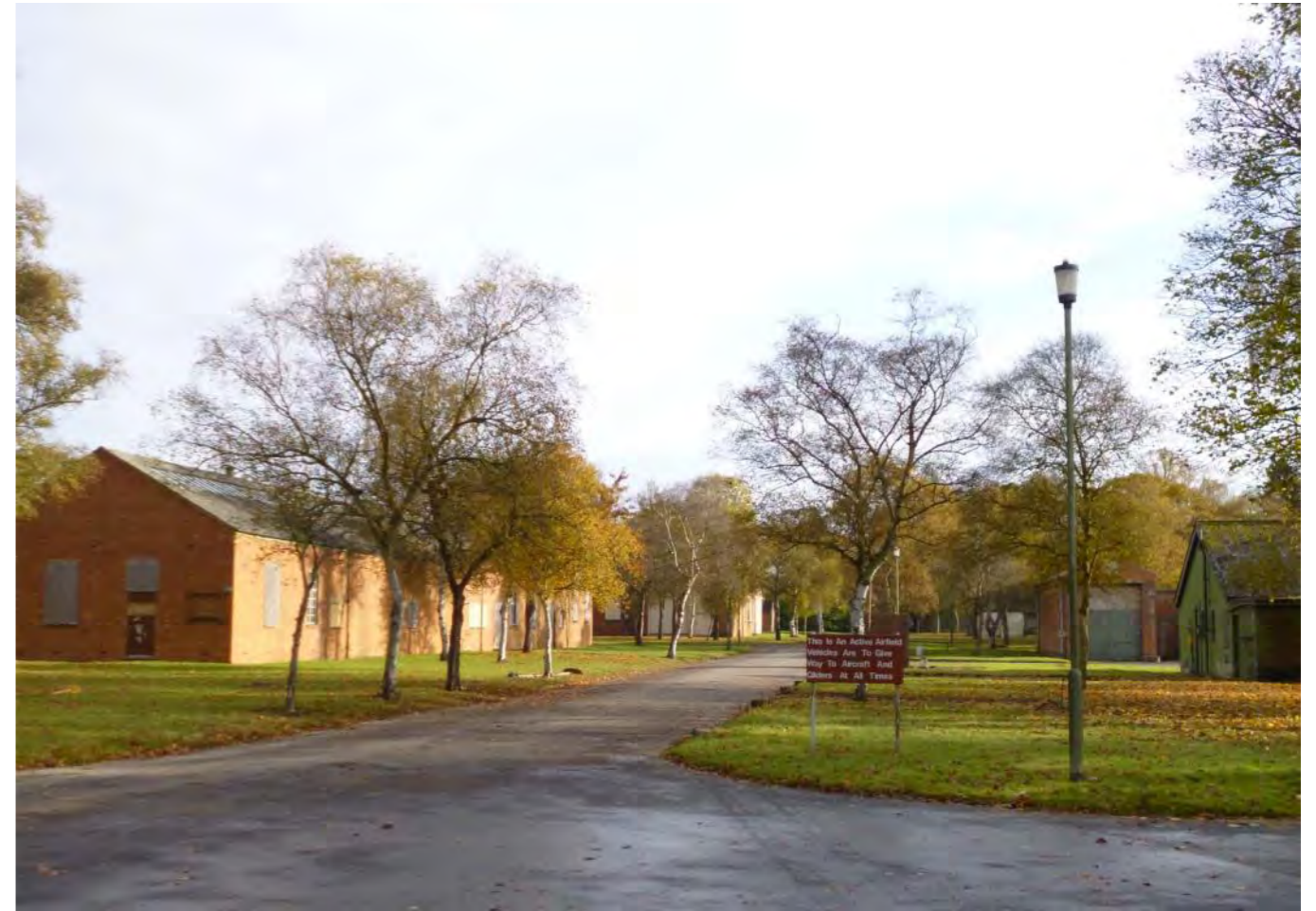
Fig 18: Approach from main entrance, Building 90 to left
