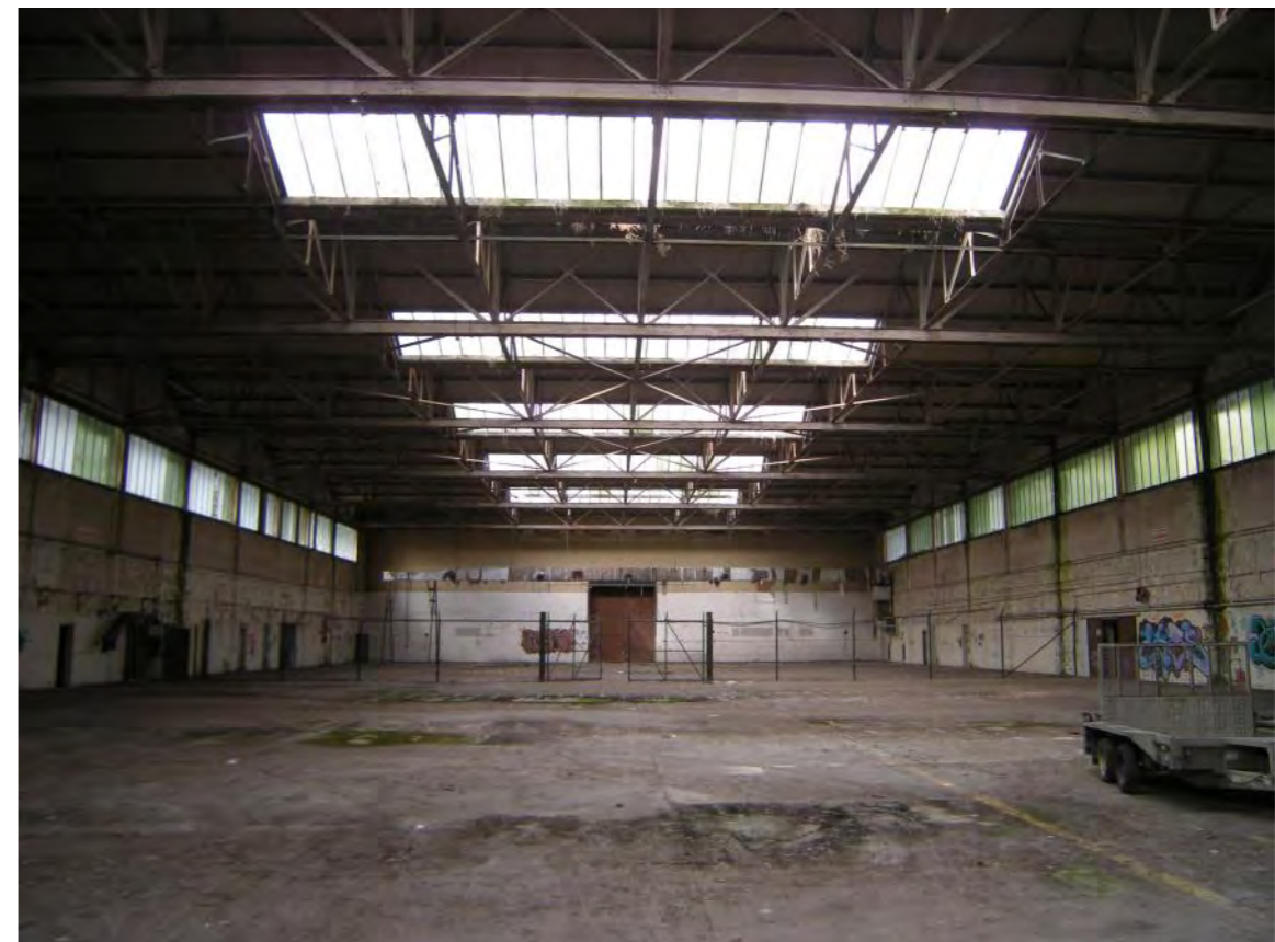
Fig 22: Interior view of Building 79
