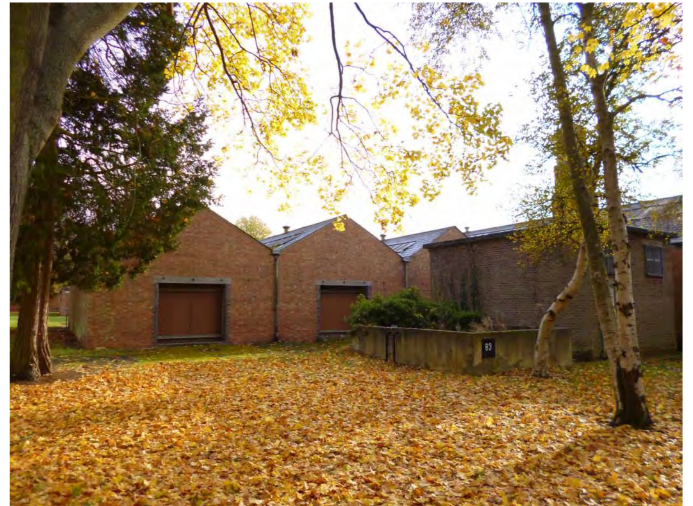
Fig 3: Building 90 from the north-west
