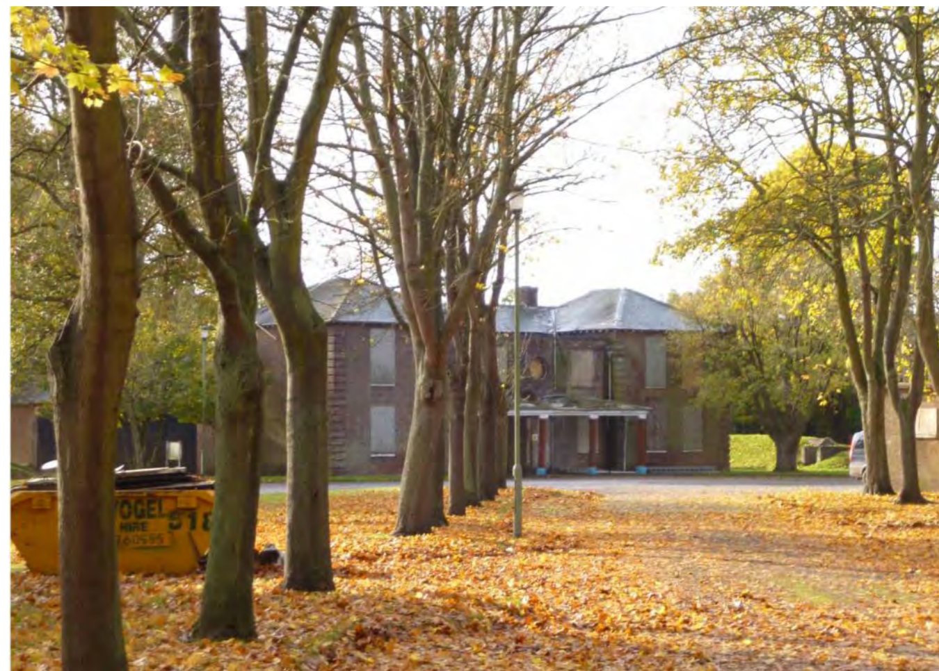
Fig 6: The Station Offices (Building 147)
