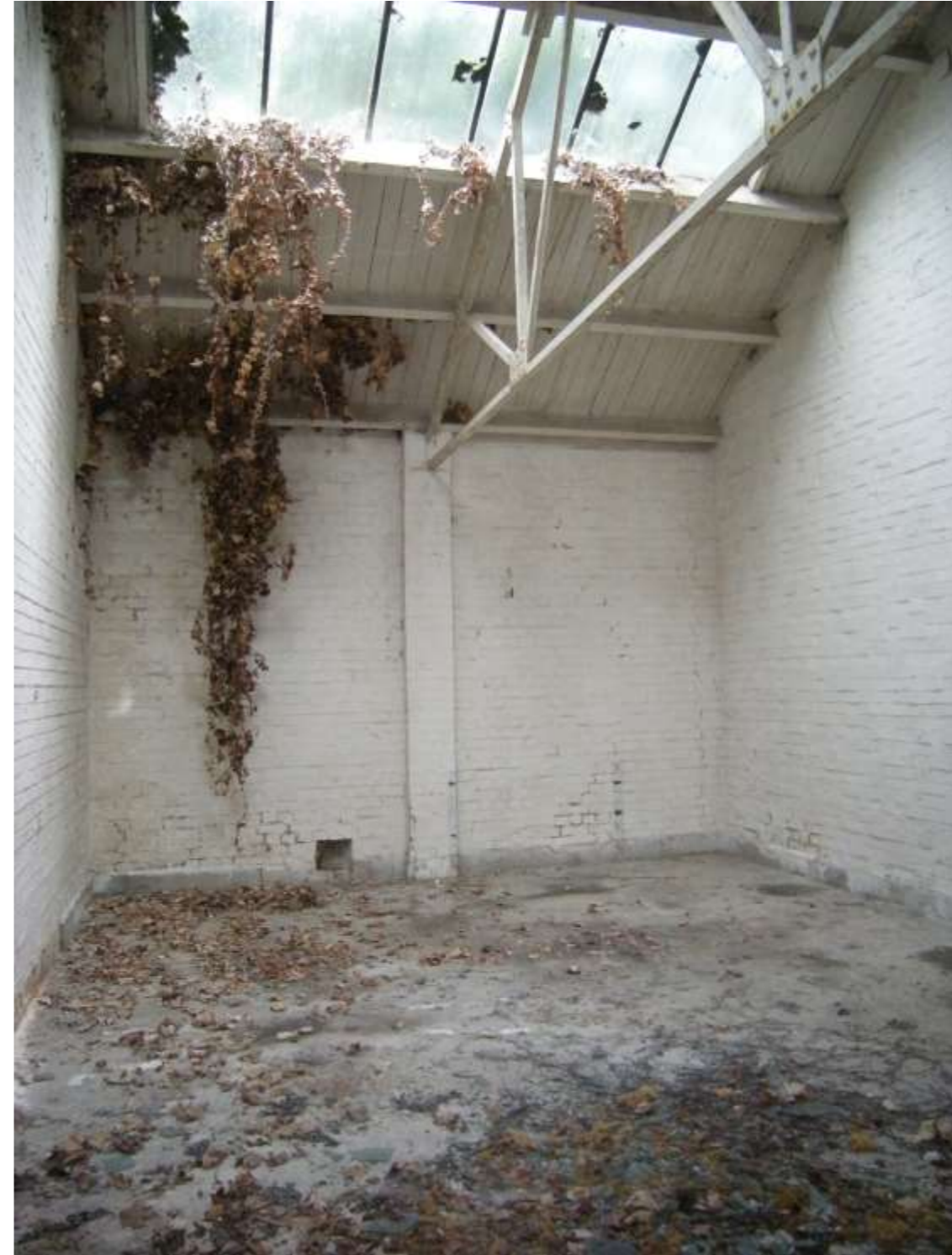
Internal view of Building 96
