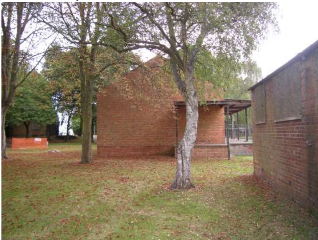
View from west of Building 96 site
