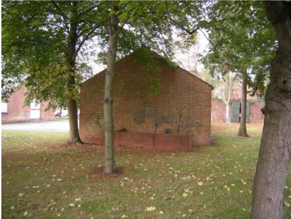
View from east of Building 96 site
