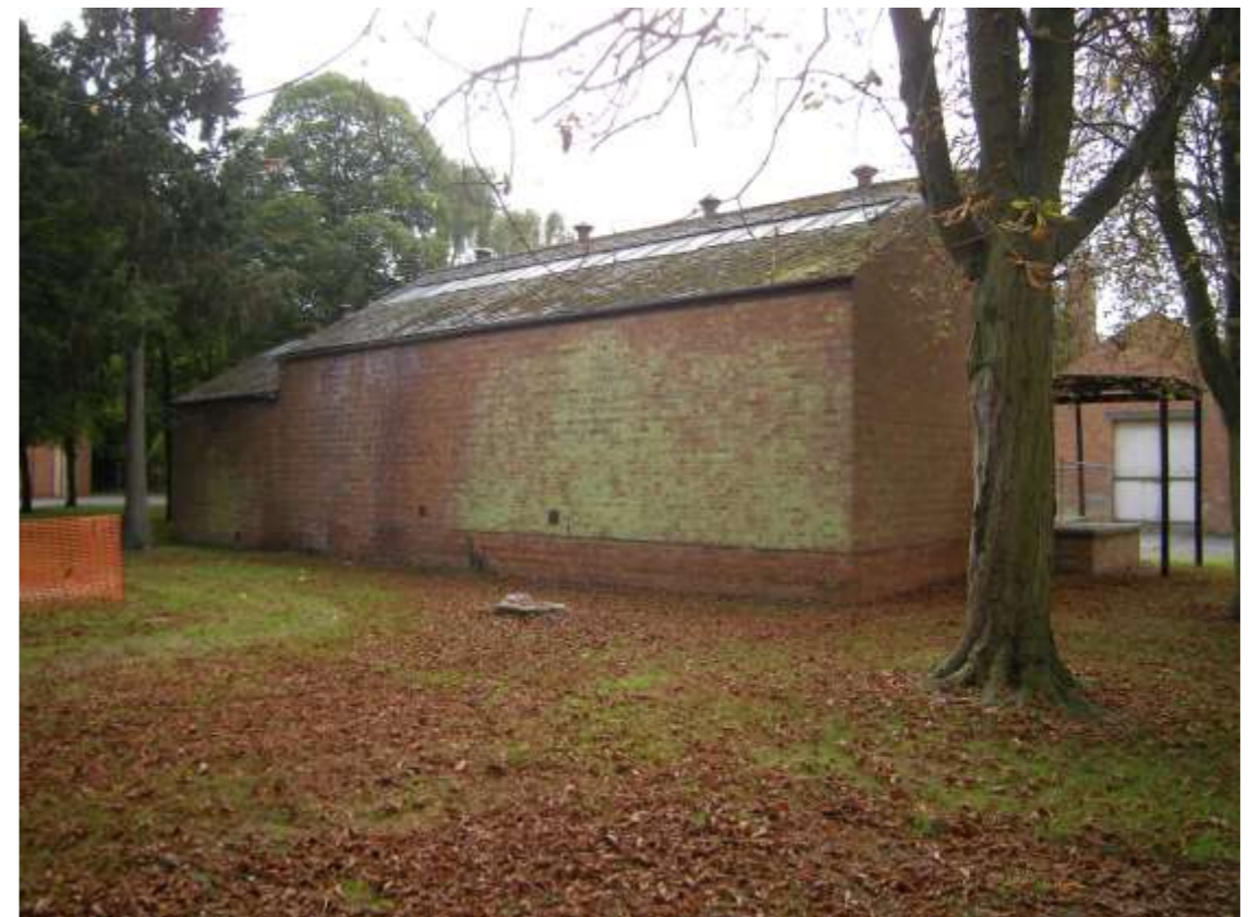
View from north of Building 96 site
