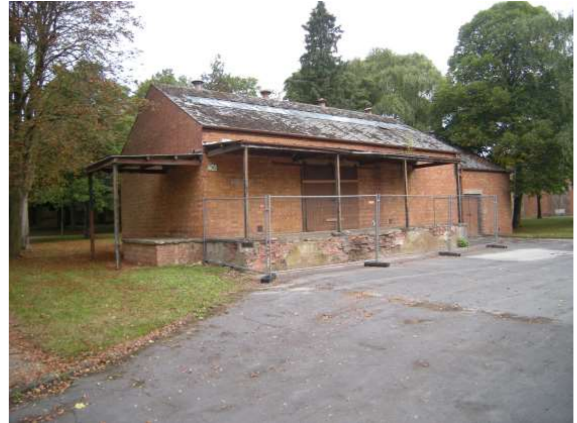
View from south of Building 96 site
