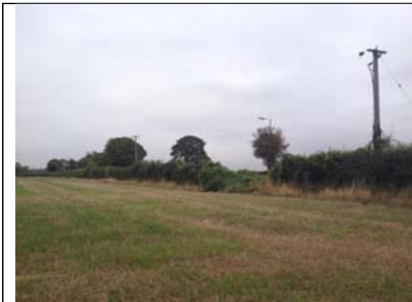
Plate 9 – Power Lines off northwest boundary
