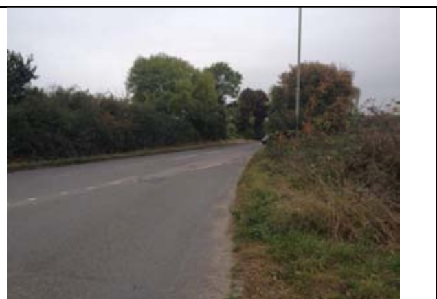
Plate 12 – Looking west along Camp Road
