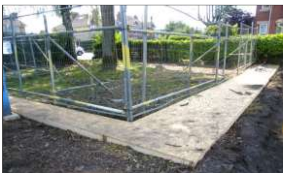
Ground protection image 3: Plywood fixed to a wood frame is another effective method of protecting soil from pedestrian compaction.
