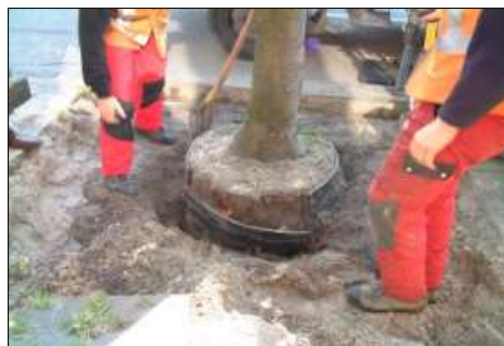
Soil cell image 4: This excavated tree shows the root deflectors that were installed when it was planted seven years previously. The product has deflected roots downwards and prevented damage to the adjacent surfacing. Note that this is a permeable sandy soil and the roots were able to grow beneath the bottom of the deflectors.
