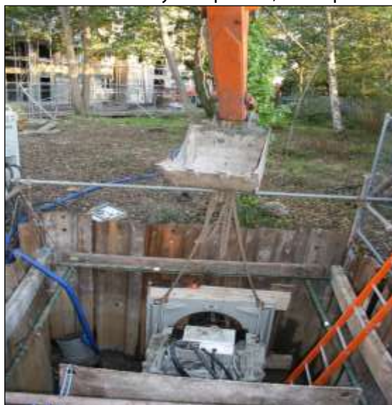
Services image 1: If possible, thrust boring is the preferred option for installing service routes through the RPAs of important trees, but there has to be space at the start and finish to dig substantial working pits.
