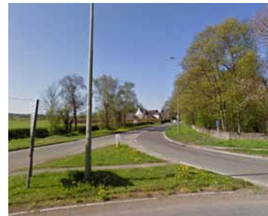
Roundabout (View on Grove Road) - Day Pole-mounted High Pressure Sodium Light (at ~ 4.5m) on Grove Road.
