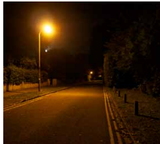
Woodstock Rd (Residential) - Night Pole-mounted High Pressure Sodium Light (at ~ 4.5m) Illuminance: 3 - 30 Lux Luminous Intensity of Light Source: 12000 cd
