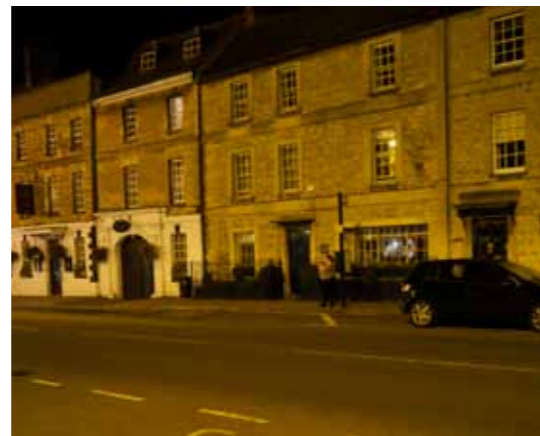
Woodstock St - Night Light trespass from wall-mounted Flood Lights on neighbouring buildings.
