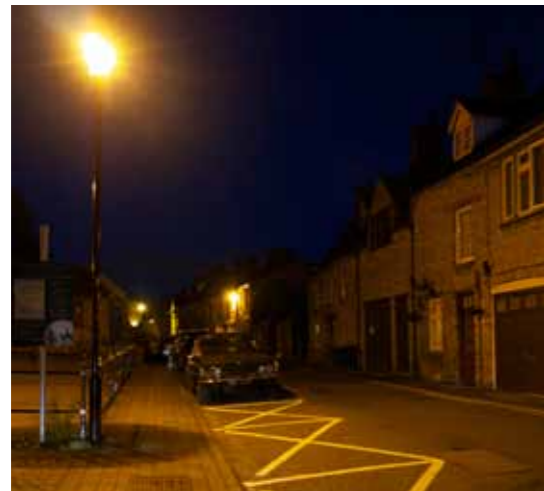
Union St - Night Pole-mounted High Pressure Sodium Light (at ~ 4.5m) Illuminance: 25 Lux Luminous Intensity of Light Source: 500 cd
