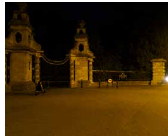
Blenheim Palace Entrance - Night Light levels from Street Lights on opposite side of the road. Illuminance: 6 Lux
