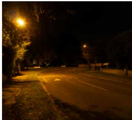
Cadogan Park - Night Pole-mounted High Pressure Sodium Light (at ~ 4.5m) Illuminance: 30 Lux Luminous Intensity of Light Source: 12000 cd
