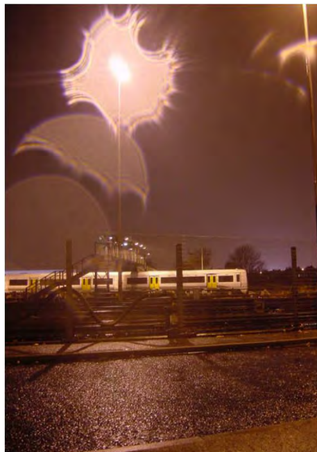
Figure 7.4 Light Spill from High Mast Luminaires
