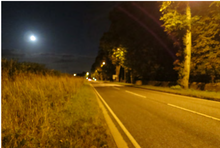
Image 7.1: A44 Oxford Road looking towards Bladon Roundabout
