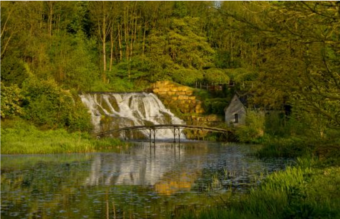
Reservoir Act compliance works to Blenheim Dam – cost £1.5m
