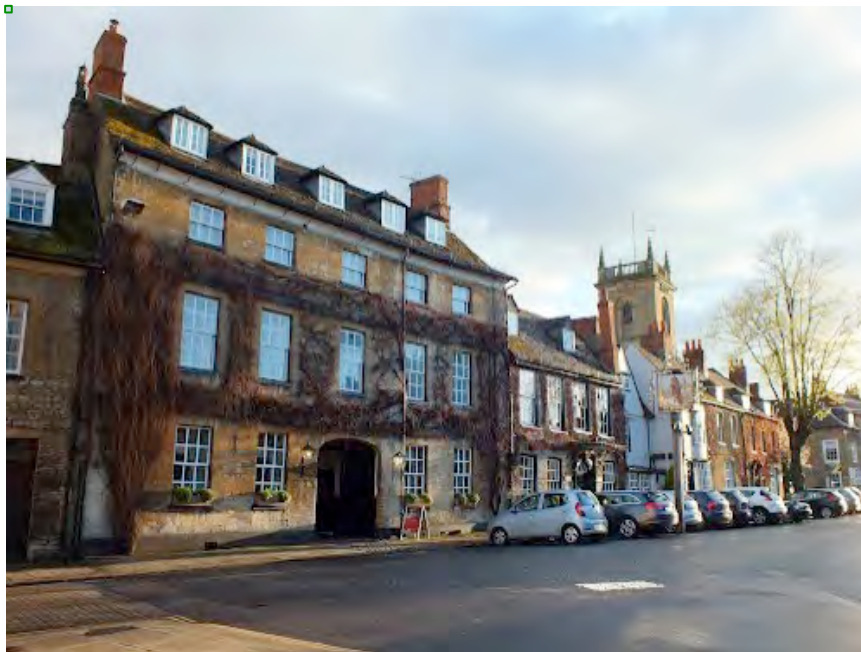
Figure 16: Existing Heritage in Woodstock High Street
