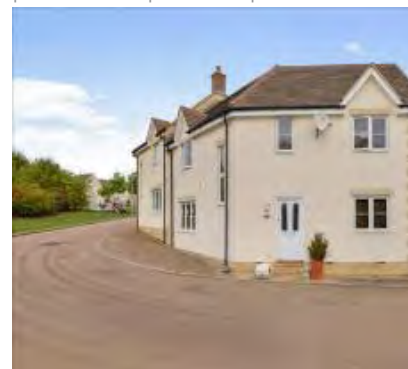
Street doesn't relate to building lines or design
