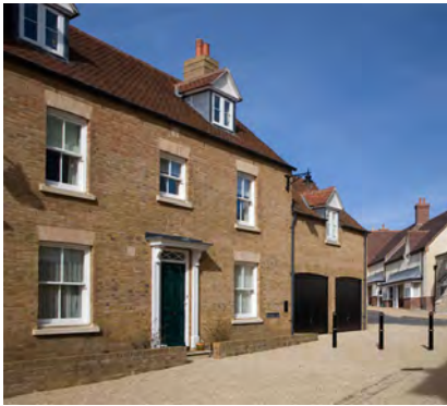
Street furniture to separate vehicle and pedestrian spaces
