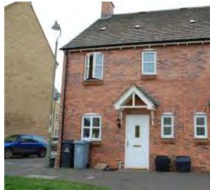
No waste storage facilities
