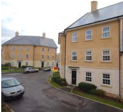
Inadequate parking provision
