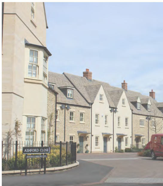
CORNER BUILDING MARKS GATEWAY
