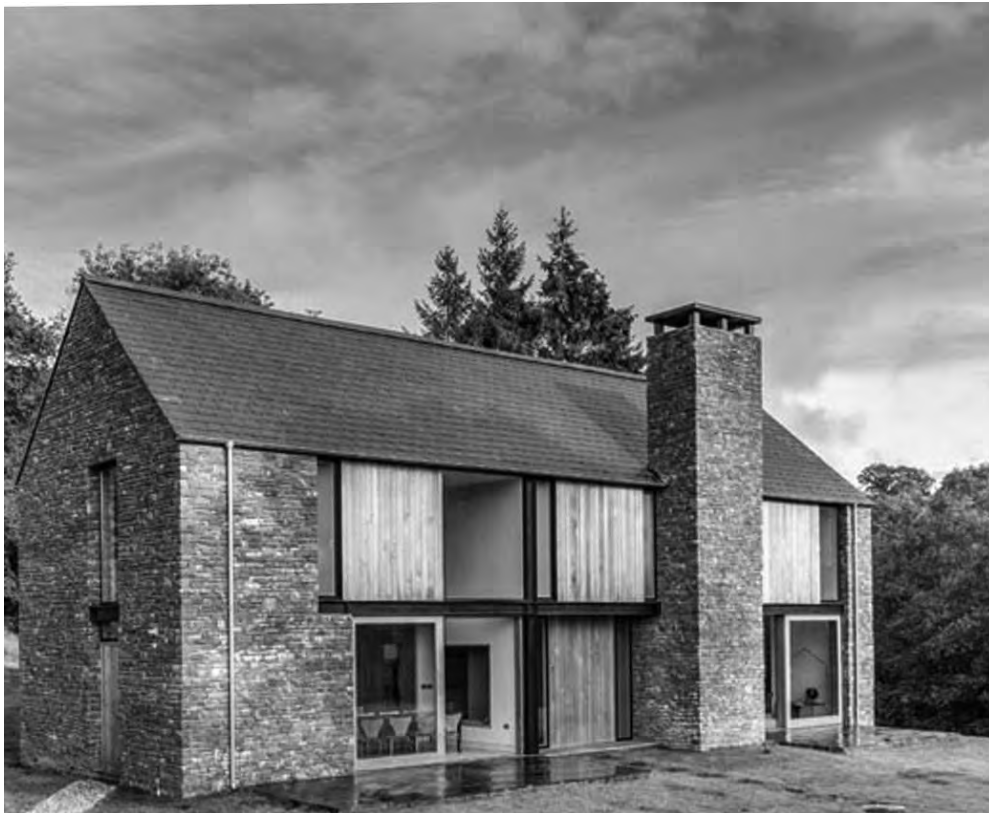
Traditional contemporary buildings
