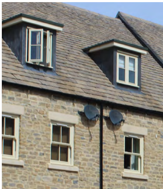
BROKEN ROOF HEIGHTS
