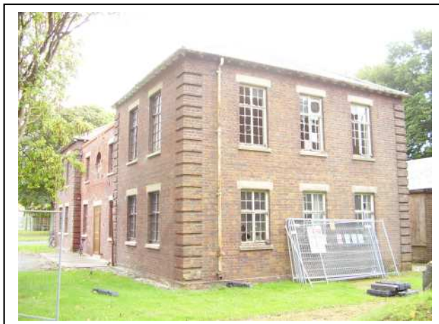
147. Large 2-Storey Brick Building
