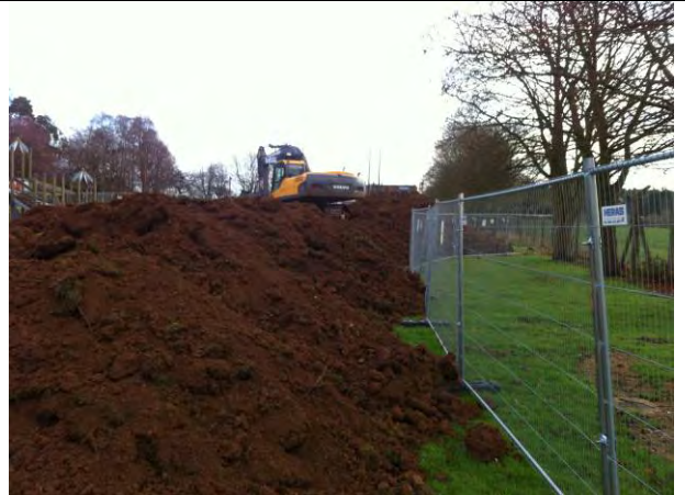
6. 18.12.13 - Phase 1A site generated topsoil
