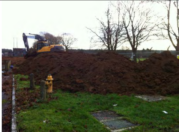
5. 18.12.13 - Phase 1A site generated topsoil
