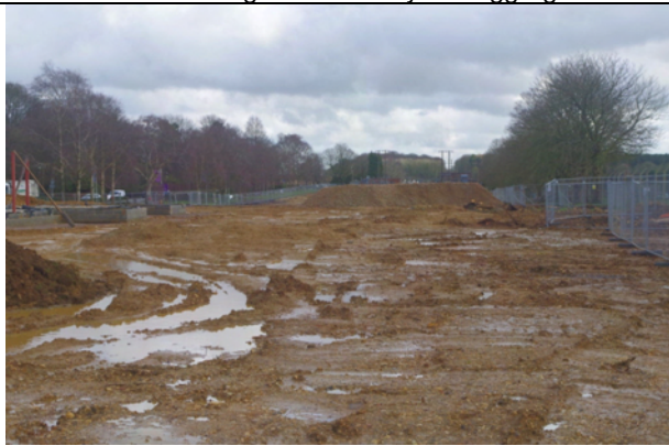
29. 25.02.14 – View from southwest facing east
