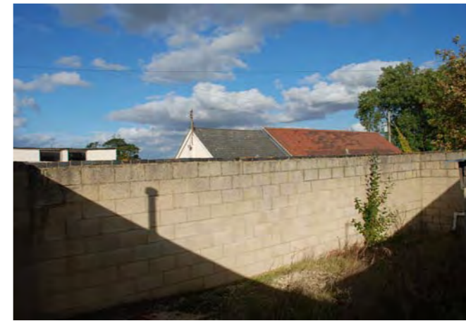
4. Boundary wall. New Barn Farm out buildings to north of wall
