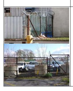
Chain link fence with concrete supports approx. 1.8m high with 45° overhang of either barbed wire strips or razor wire strips.
