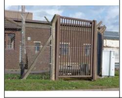
W Galvanised chain link approx. 2.50m high with concrete supports topped with a 45° overhang with strips of barbed wire.
