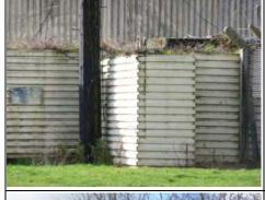
Metal construction  $\circ$ blast wall structure. approx. 2.25m high and no overhang.
