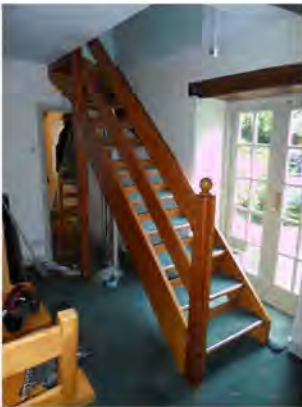
2.4 Stair to be removed
