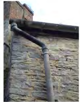
4.1 Asbestos gutters replaced
