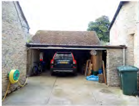
5.1 Flank wall to be removed
