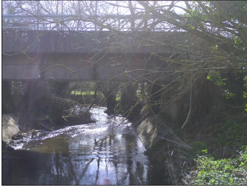
Figure 8 – Upstream Face of Railway Bridge Modelled as USBPR Bridge Unit at ISIS node LB2.
